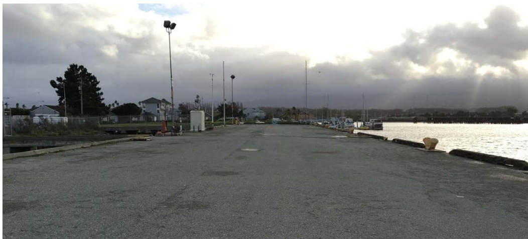
Figure 61: View on Wharf 5 looking south/west. The pier is well maintained, wide, structurally sound, and available.
