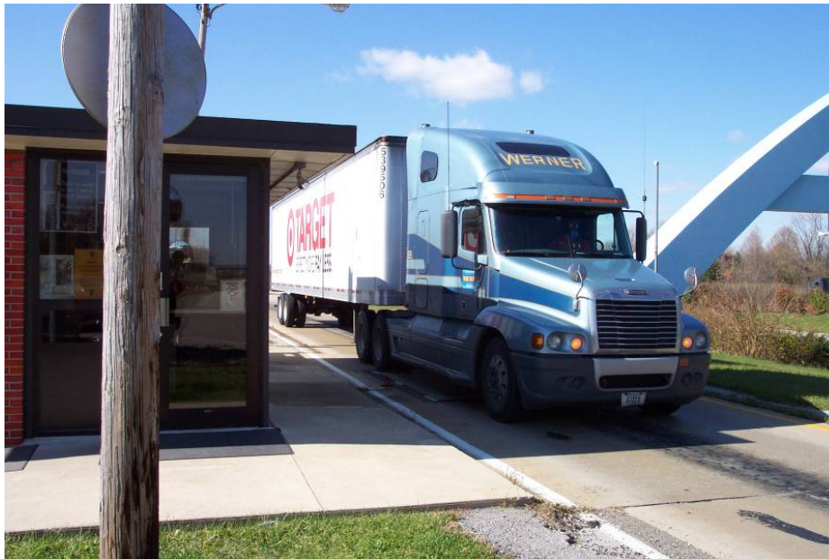
Figure 7-2. Preble County Scale House, Eaton, Ohio
