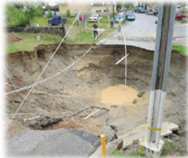
Permanent Repair Work
