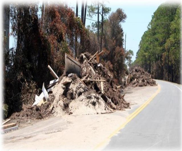
Emergency Repair Work
