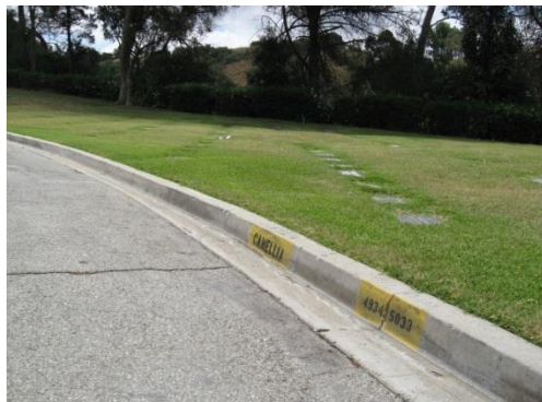
Figure 4.54: Barrier Curb / No Shoulder (Code ‘7’)
