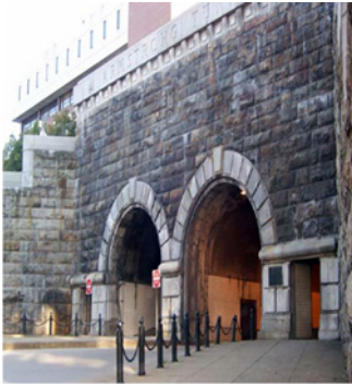
Figure 4.10: Tunnel (Code ‘2’) Example
