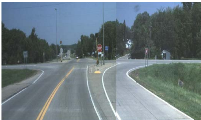
Figure 4.42 Stop Sign Controlled Intersection
