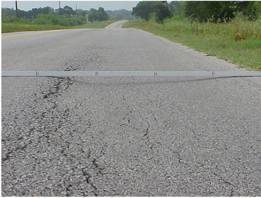
Figure 4.72 Rutting Example
