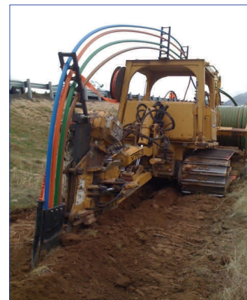
Conduit being installed along I-80 in Utah.
