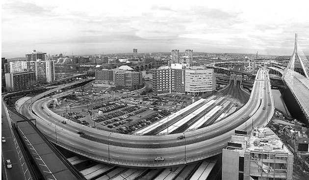
Overview of construction at the Central Artery/Tunnel Project in Boston.
