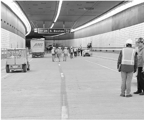
“Big Dig” tunnel in Boston.
