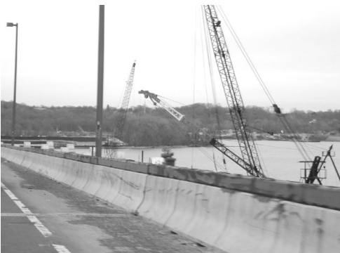
Woodrow Wilson Bridge construction.
