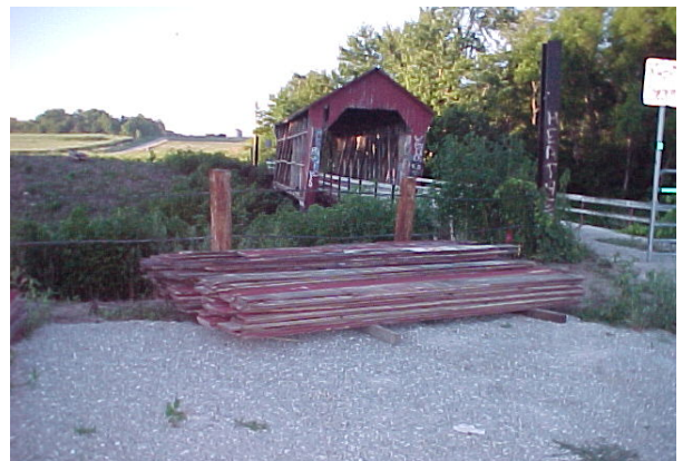
Figures 35 & 36 Removing and storing siding.
