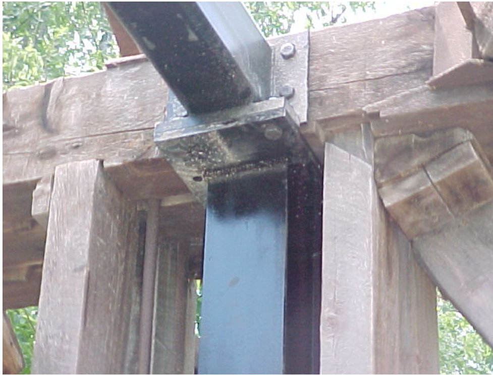
Figure 27 Steel bolted to the historic timber.
