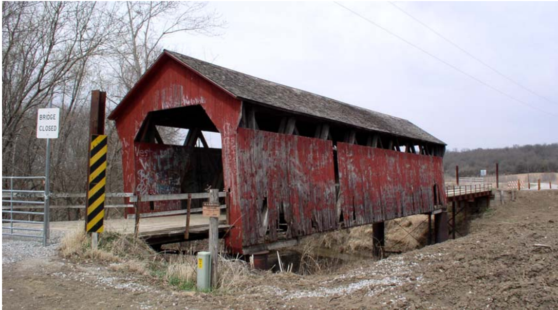
Figure 8 Hammond Bridge just prior to its rehabilitation in April 2003. (Nash photo)
