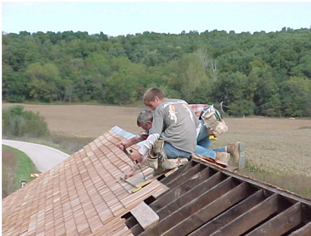
Figure 40 Re-roofing with cedar shingles.
