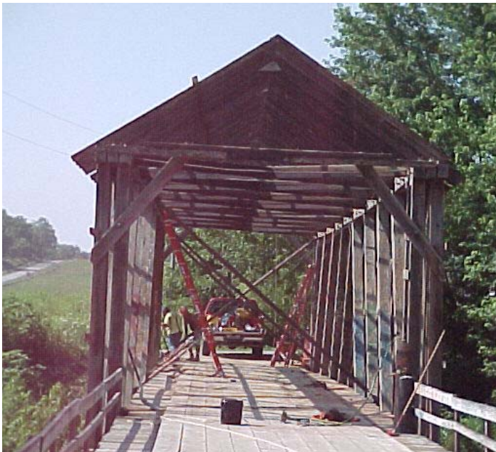
Figures 16 and 17 Straightening the trusses, looking south. (Drawing adapted from Shuck-Britson Inc. rehabilitation plans dated January 2003; Jay Davis photo on left)
