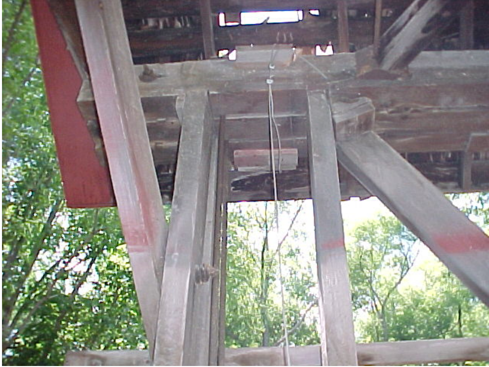
Figure 22 The steel was installed in the space between timber uprights.
