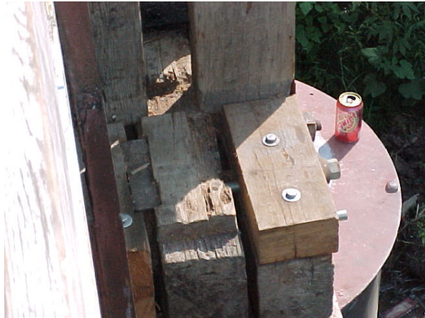
Figures 30 & 31 Floor beam and pier trouble spots.
