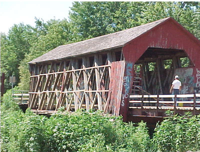
Figures 35 & 36 Removing and storing siding.
