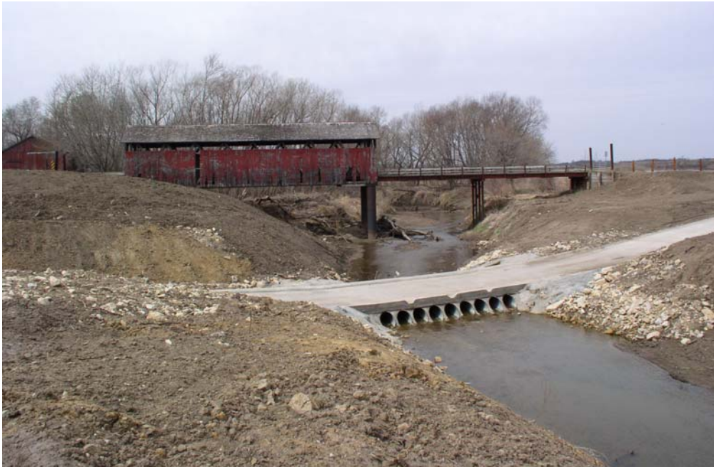
Figure 19 A new concrete ford just downstream from Hammond Bridge now carries the road's vehicular traffic and a small pull-out at the north end of the approach (to the right) provides graveled parking for several cars. (Nash photo)
