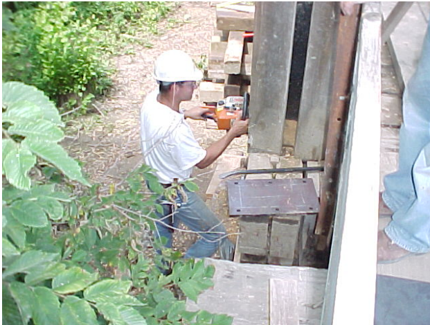
Figures 23 & 24 Setting the foot plate for the steel.
