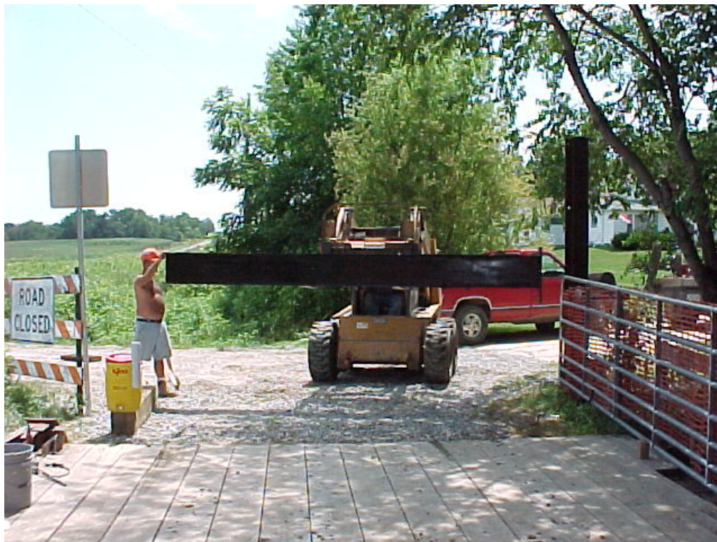
Figure 25 Bringing steel for the new portal beam.
