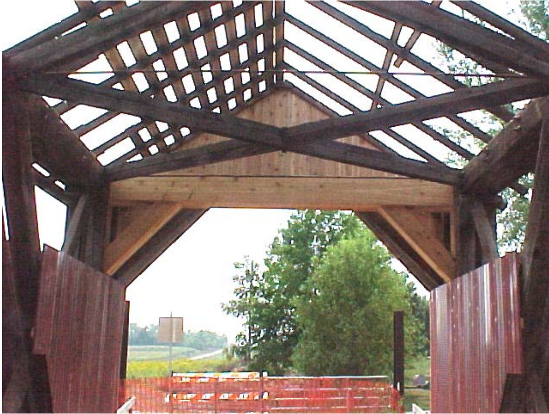
Figure 29 The reinforced southern portal, clad in new cedar.
