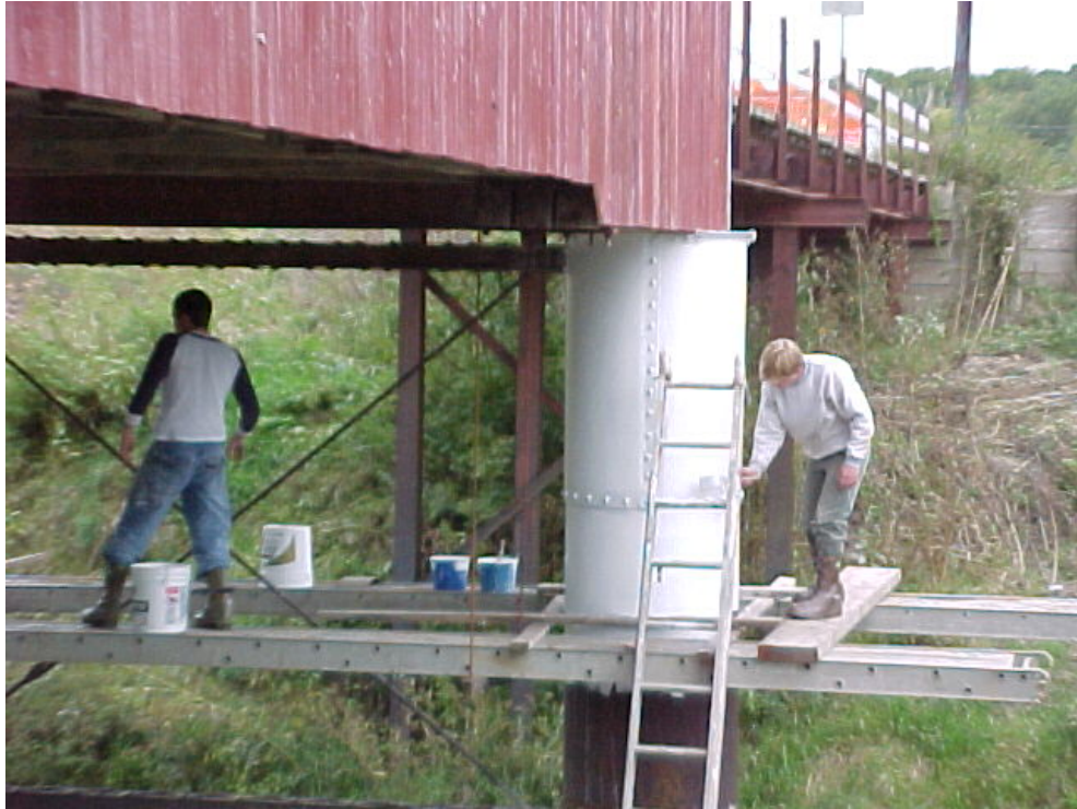
Figure 33 Priming a caisson/cylinder pier.
