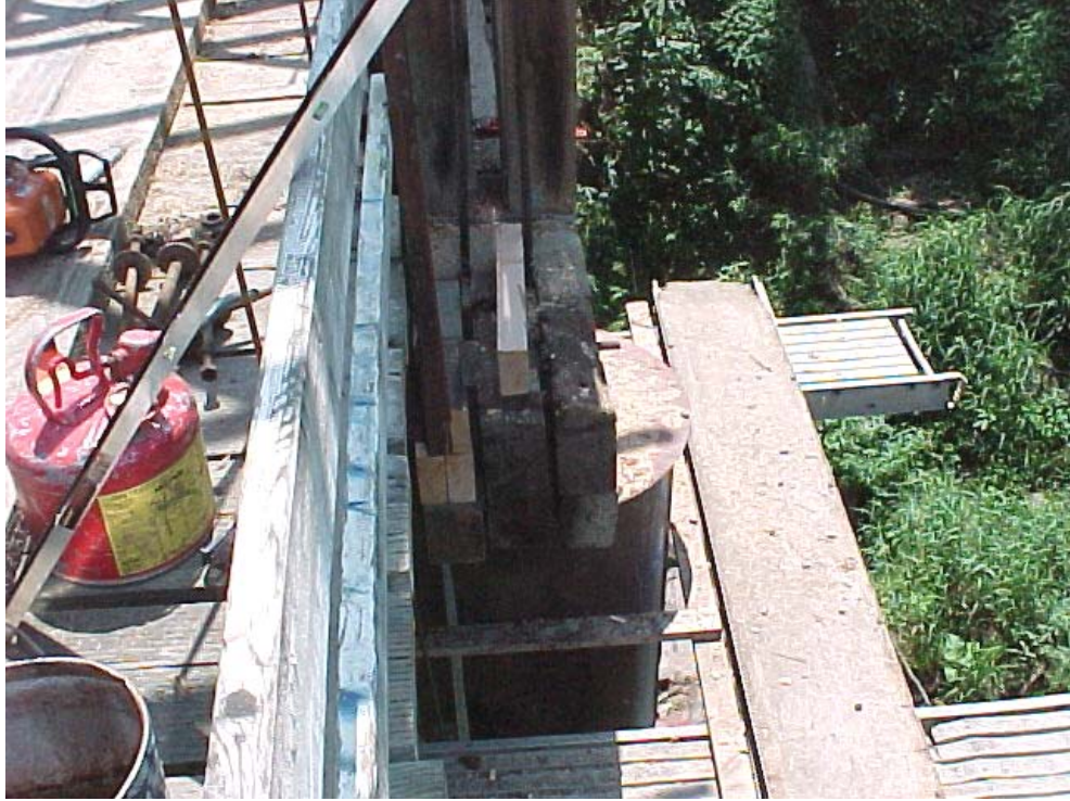
Figure 32 Repairing the rotten wood at the northwest caisson area.
