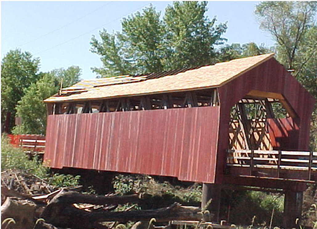
Figure 39 The roofing in process.
