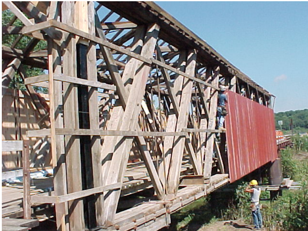
Figure 38 Replacing the siding.
