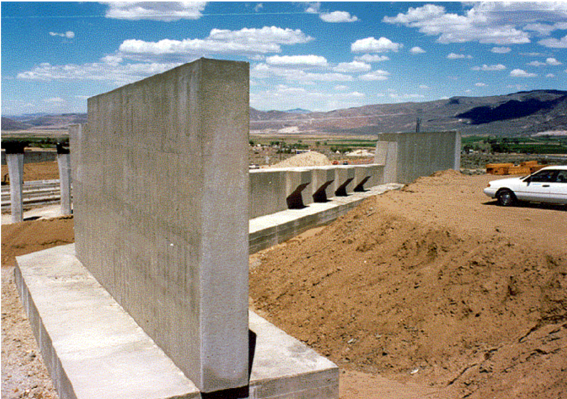
Figure 2-14: Footing at South Abutment, I-580, Nevada
