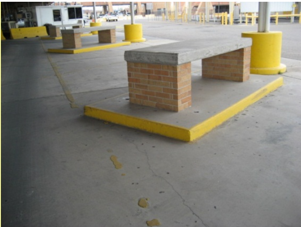
Above: Hidalgo, TX. This is clearly an inadequate passenger waiting area. Up to 3 buses may be inspected at one time, posing a safety and security concern for both FMCSA personnel and the numerous bus passengers.
