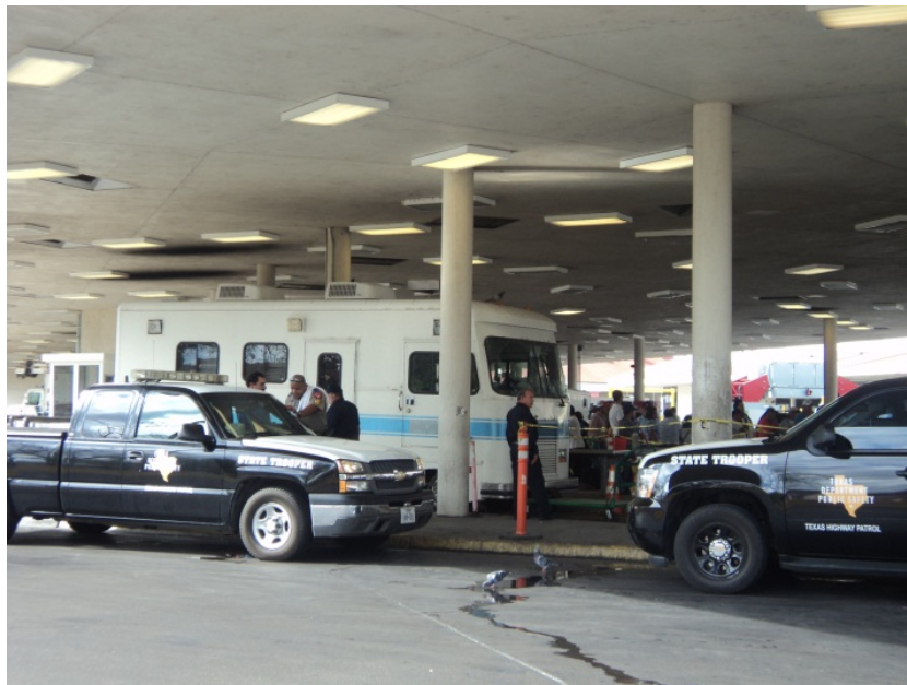
Above: This photo shows the total lack of bus inspection facilities at Laredo (Lincoln-Juarez). This facility is always extremely busy and we have no way of controlling off-loaded passengers during our inspection process. This increases inspection times for buses and opens us up to passenger safety issues if the bus is placed out of service. The camper in the picture is used as the agency's temporary working space. The off-loaded passengers can be seen in the back of the picture. This is an example where there is at least a canopy for the passengers but no place for them to sit while they wait for a bus to pick them up again and bring them to their destination. Their bus was placed out of service.
