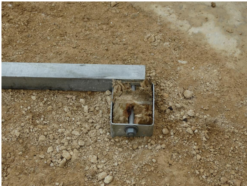
Figure 3.9: Post Test – Foundation Sleeve at Post 1
