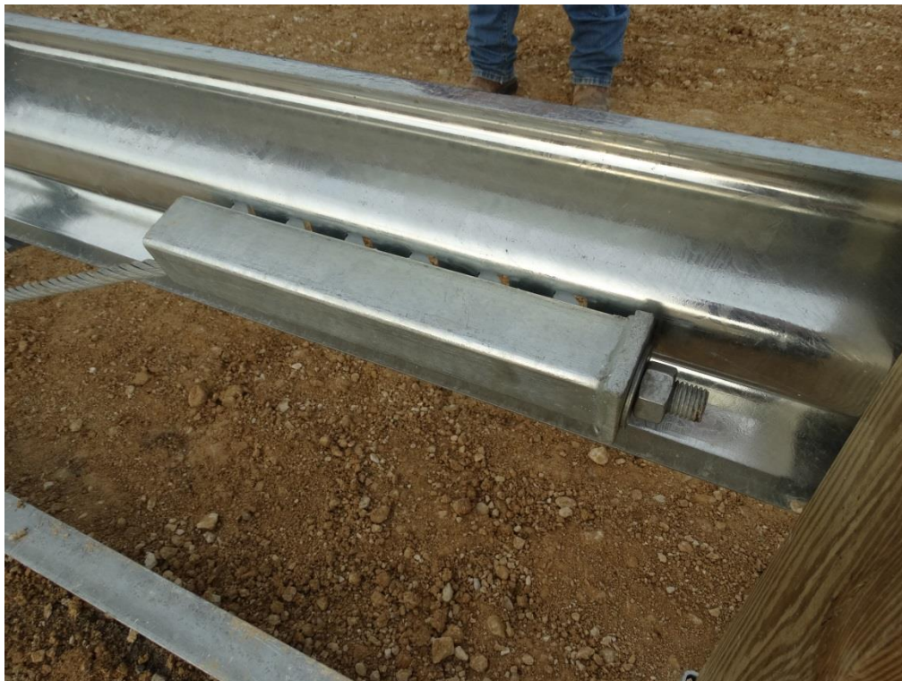
Figure 2.10: End Terminal Cable Anchor at Downstream End
