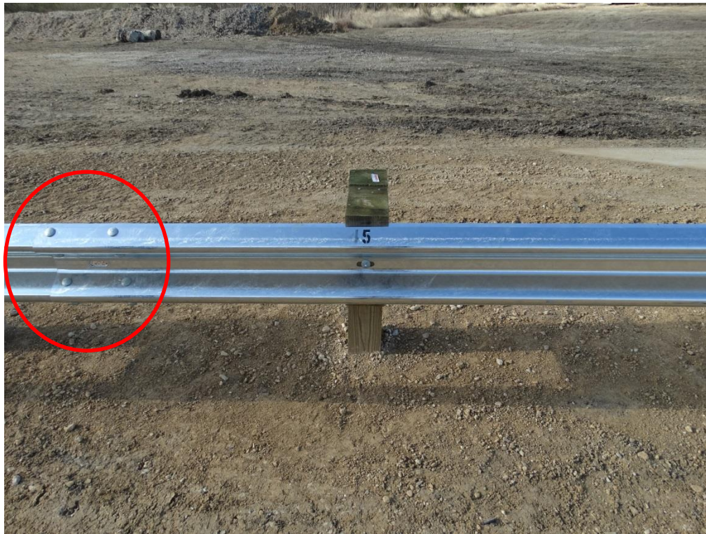
Figure 2.13: Second Guardrail Panel Splice Joint Mid-Span between Posts 5 & 6 – Traffic Side
