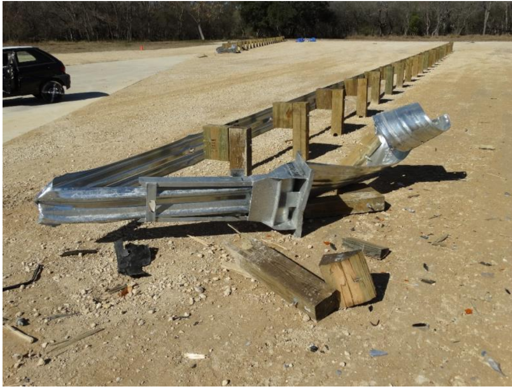
Figure 3.46: Post Test – Traffic Side View of Gated End Terminal
