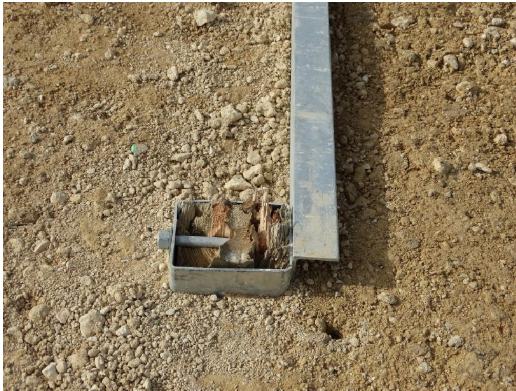
Figure 3.13: Post Test – Foundation Sleeve at Post 1
