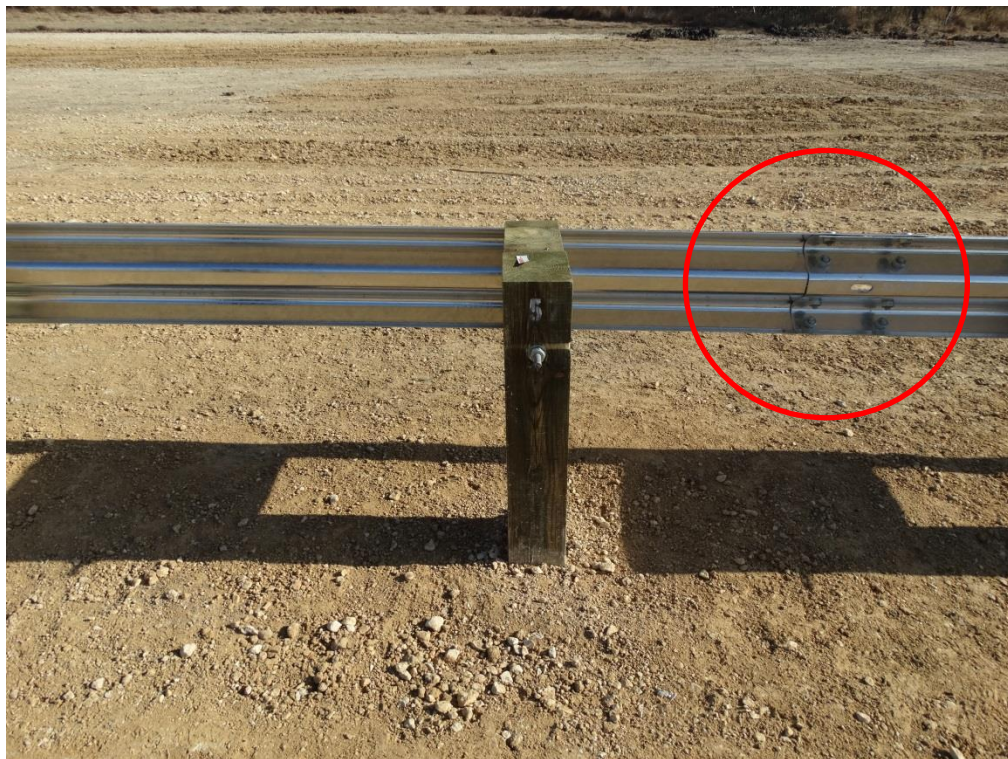
Figure 2.14: Second Guardrail Panel Splice Joint Mid-Span between Posts 5 & 6 – Non-Traffic Side
