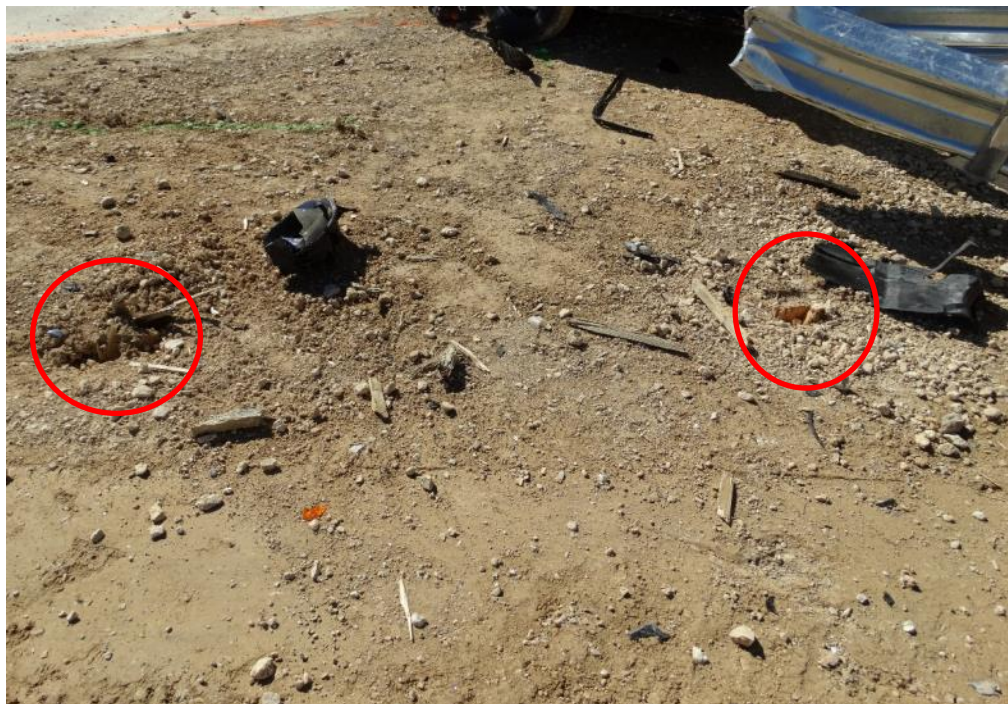
Figure 3.18: Post Test – Non-Traffic View of Post 3 (Left) and Post 4 (Right)
