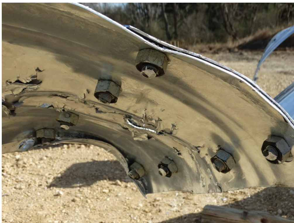
Figure 3.23: Post Test – Extruded Guardrail Splice from Post 3 (Splice Nuts Painted Pre-Test for Visibility in Video)
