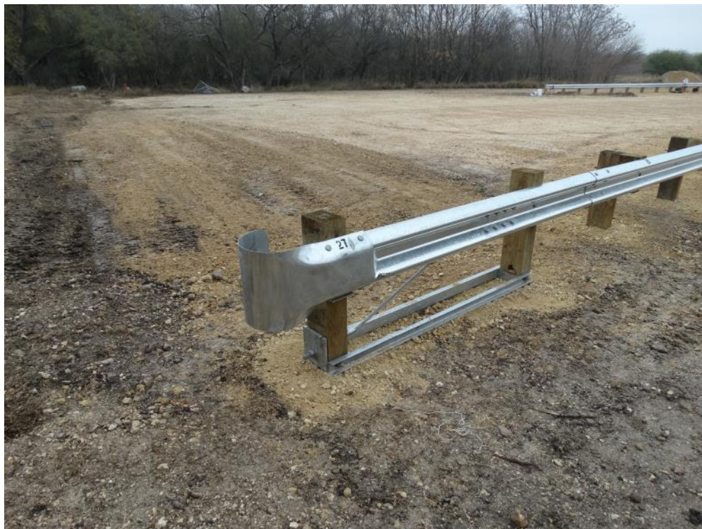
Figure 2.18: Downstream Anchor Terminal at Posts 26 and 27 – Traffic Side
