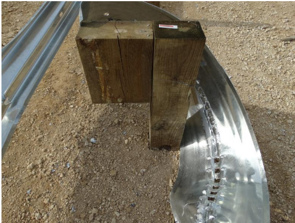
Figure 3.23: Post Test – Side View of Post 6
