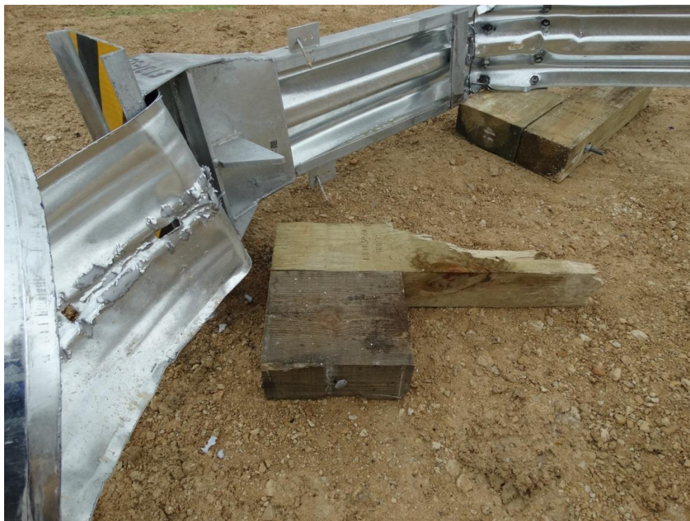
Figure 3.29: Post Test – Non-Traffic Side of Guide Channels
