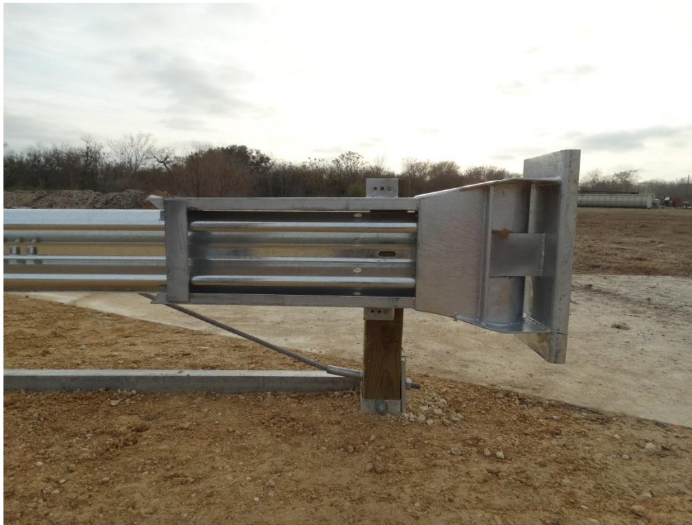
Figure 2.15: ET Plus Head and Post 1 – Traffic Side
