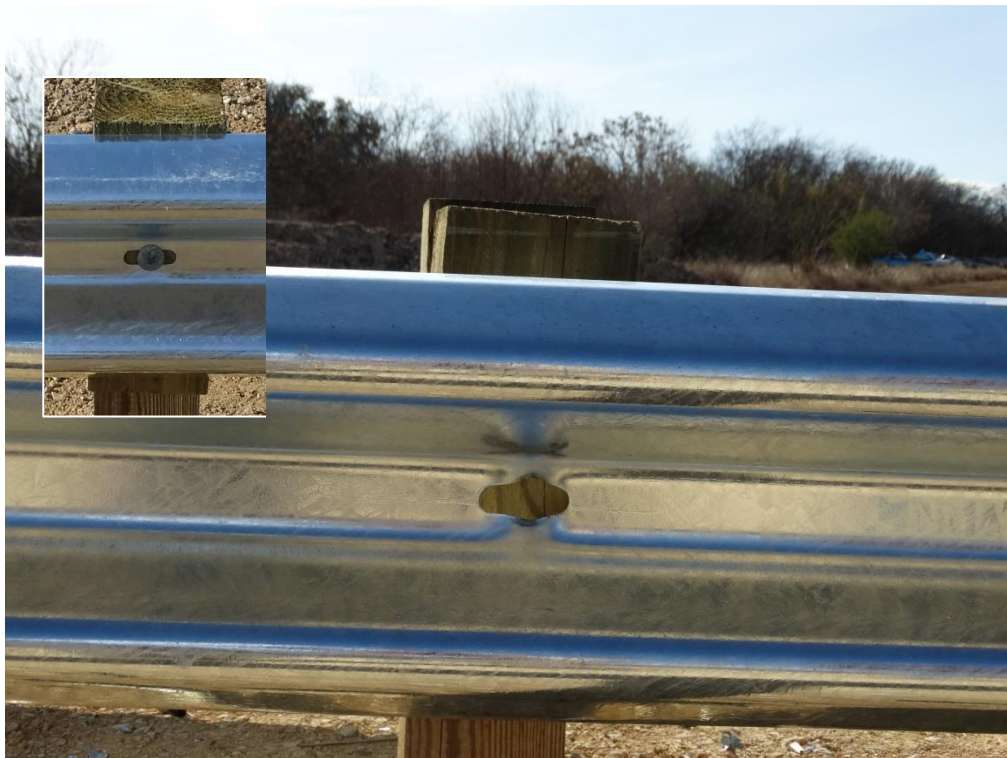
Figure 3.15: Post Test – Post 10, W Beam Pulled off Blockout (Pre-Test Photo Inset)
