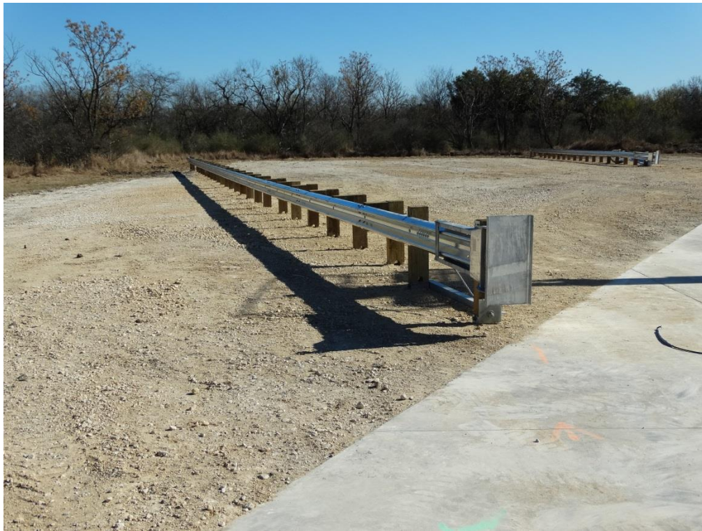
Figure 2.3: Test Installation for ET Plus Test ET31-32
