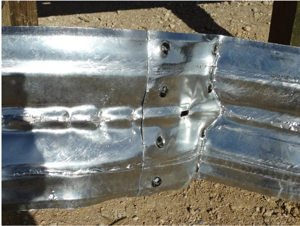
Figure 3.26: Post Test – Extruded Guardrail Splice from between Posts 7 & 8 (Splice Bolts Painted Pre-Test for Visibility in Video)
