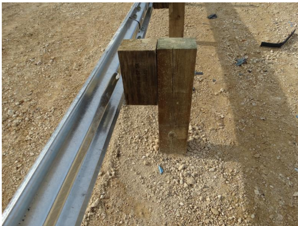
Figure 3.29: Post Test – Side View of Post 9
