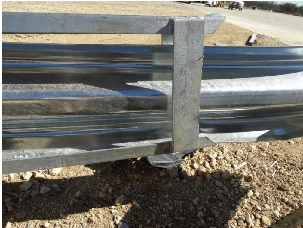
Figure 3.42: Post Test – Non-Traffic Side View of Guide Channel Entrance
