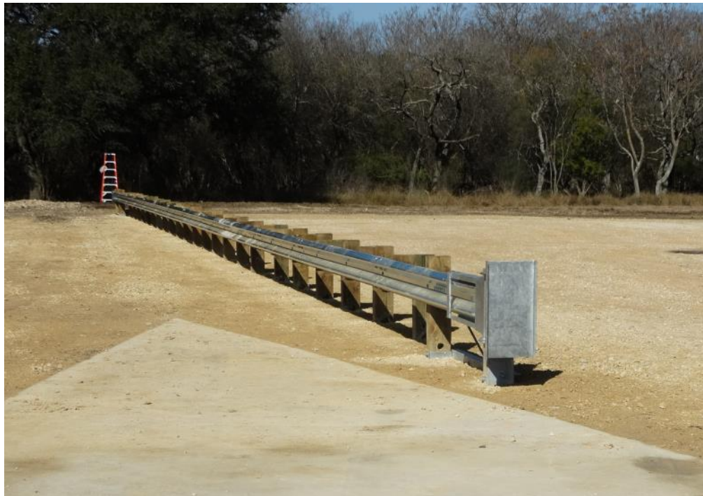
Figure 2.3: Test Installation for ET Plus Test ET31-33
