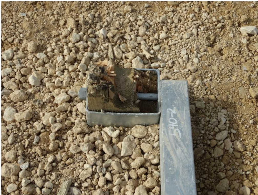
Figure 3.14: Post Test – Foundation Sleeve at Post 2
