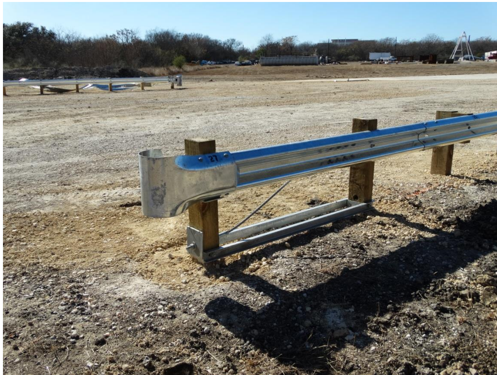
Figure 2.19: Downstream Anchor Terminal at Posts 26 and 27 – Traffic Side
