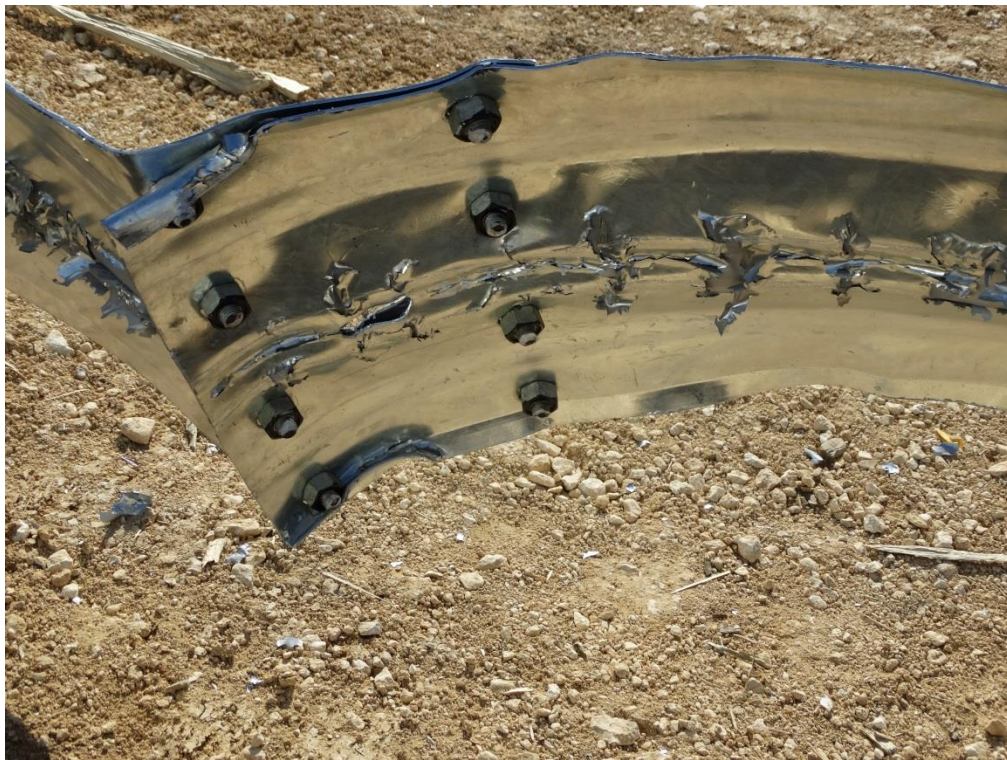
Figure 3.27: Post Test – Extruded Guardrail Splice from between Posts 7 & 8 (Splice Nuts Painted Pre-Test for Visibility in Video)
