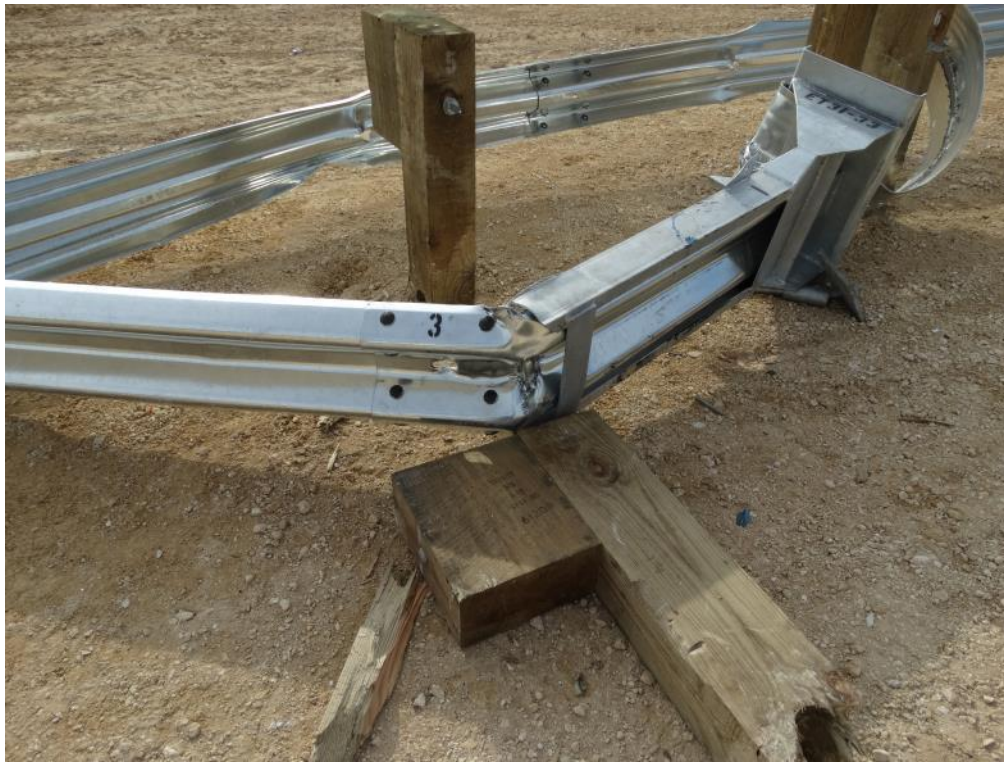
Figure 3.9: Post Test – Traffic Side of Guide Channel Entrance (Post 4 in Foreground)
