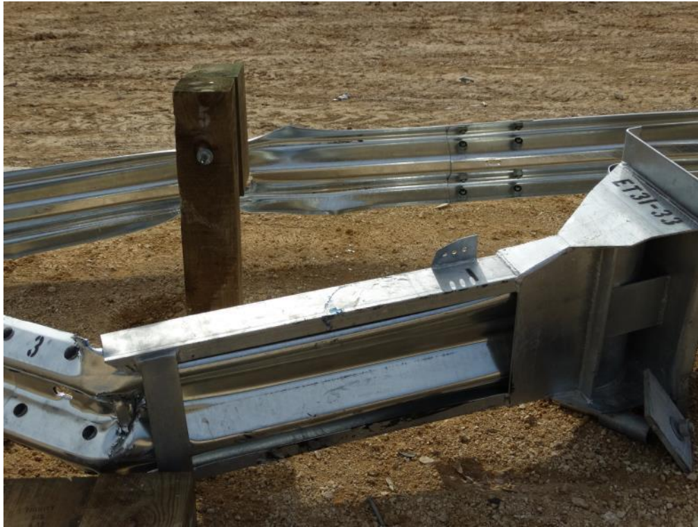
Figure 3.31: Post Test – ET Plus Head Guide Channels, Traffic Side
