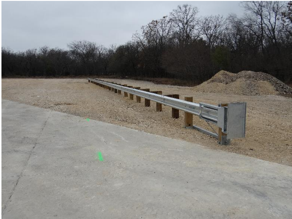
Figure 2.3: Test Installation for ET Plus Test ET31-30
