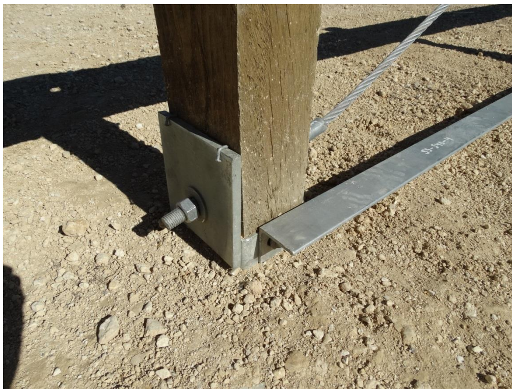
Figure 2.9: End Terminal Cable Anchor at Upstream End – Post 1
