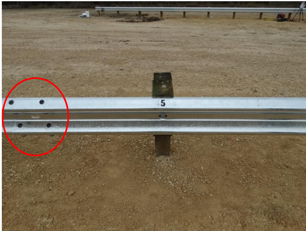
Figure 2.13: Second Guardrail Panel Splice Joint Mid-Span between Posts 5 & 6 – Traffic Side (Splice Bolts Painted for Visibility in Video)
