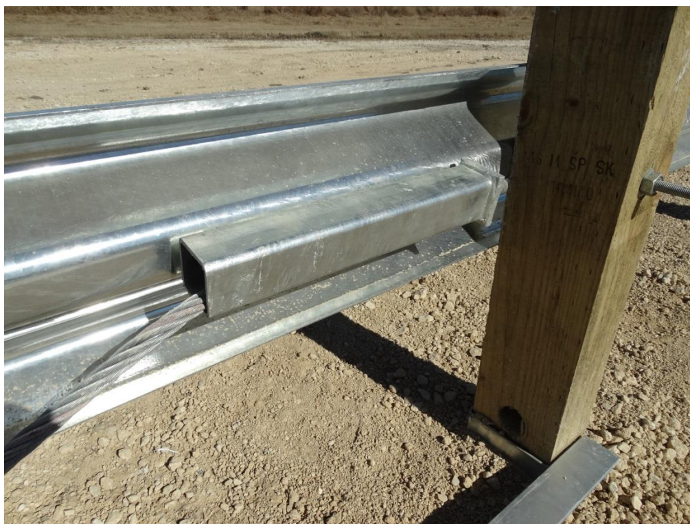
Figure 2.10: End Terminal Cable Anchor at Downstream End
