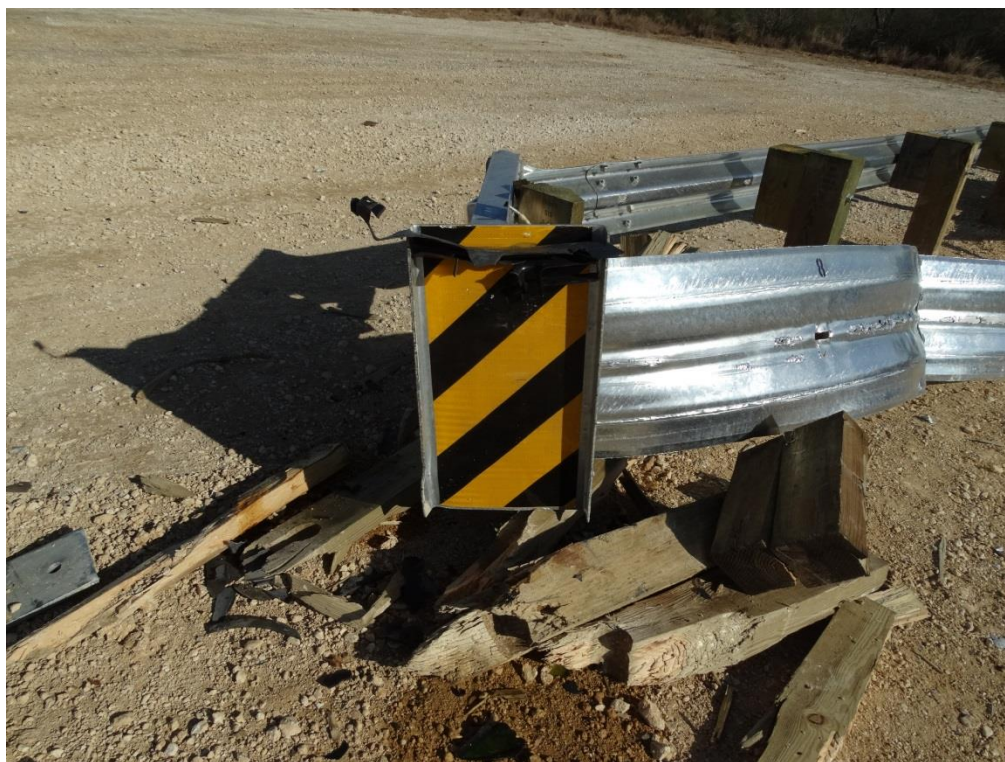
Figure 3.40: Post-Impact Test Article after Vehicle Removed – Impact Plate
