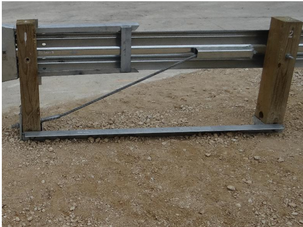
Figure 2.8: ET Plus Head and Anchor Cable Assembly
