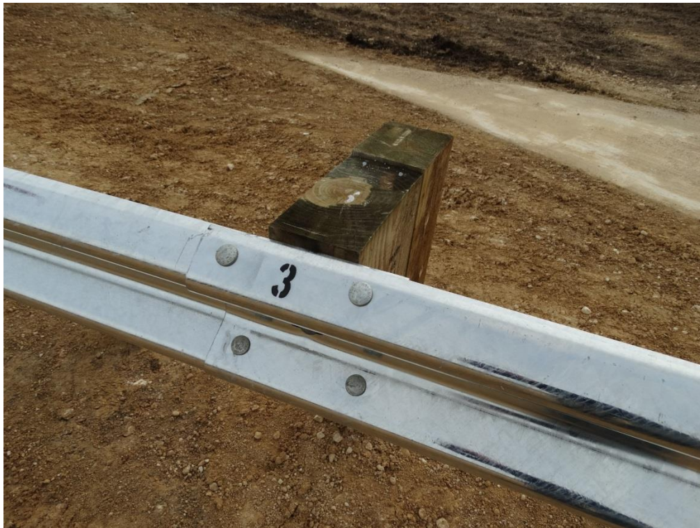
Figure 2.11: First Guardrail Panel Splice Joint – Traffic Side
