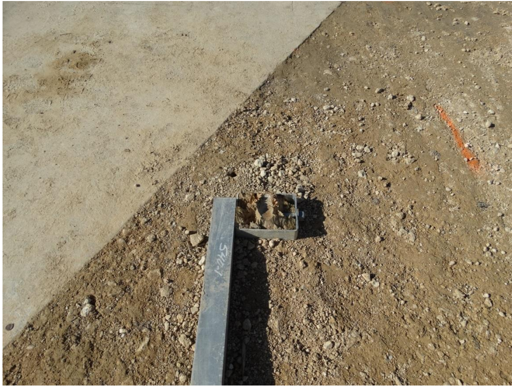
Figure 3.8: Post Test – Post 1 Foundation Sleeve
