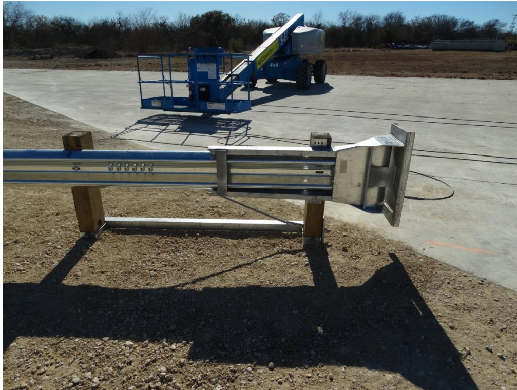
Figure 2.17: End Terminal Head with Posts 1 & 2 and Strut
