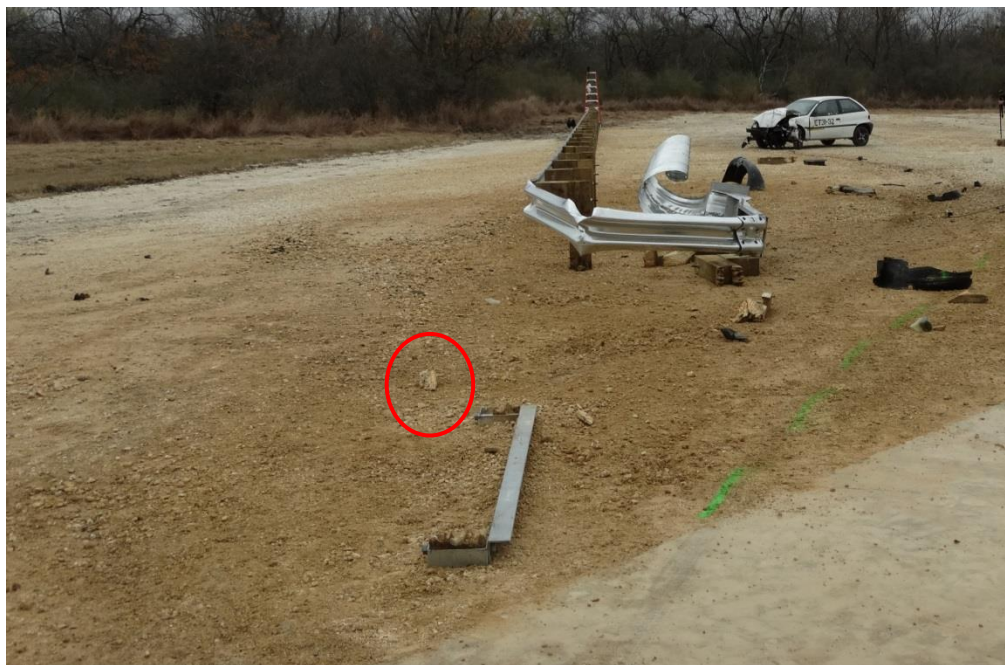
Figure 3.34: Post Test – Debris on Traffic Side
