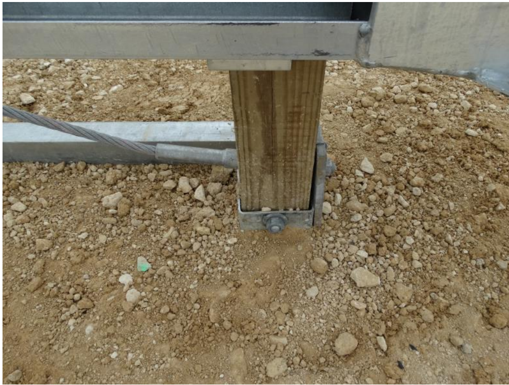
Figure 2.9: End Terminal Cable Anchor at Upstream End – Post 1
