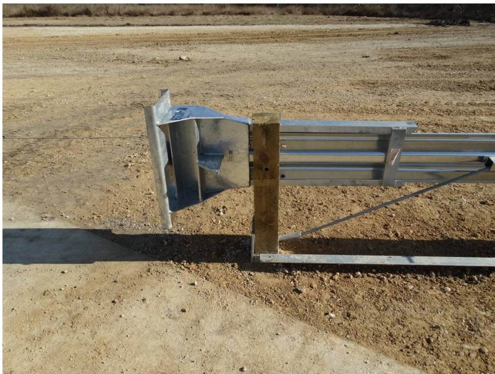
Figure 2.16: ET Plus Head and Post 1 – Non-Traffic Side
