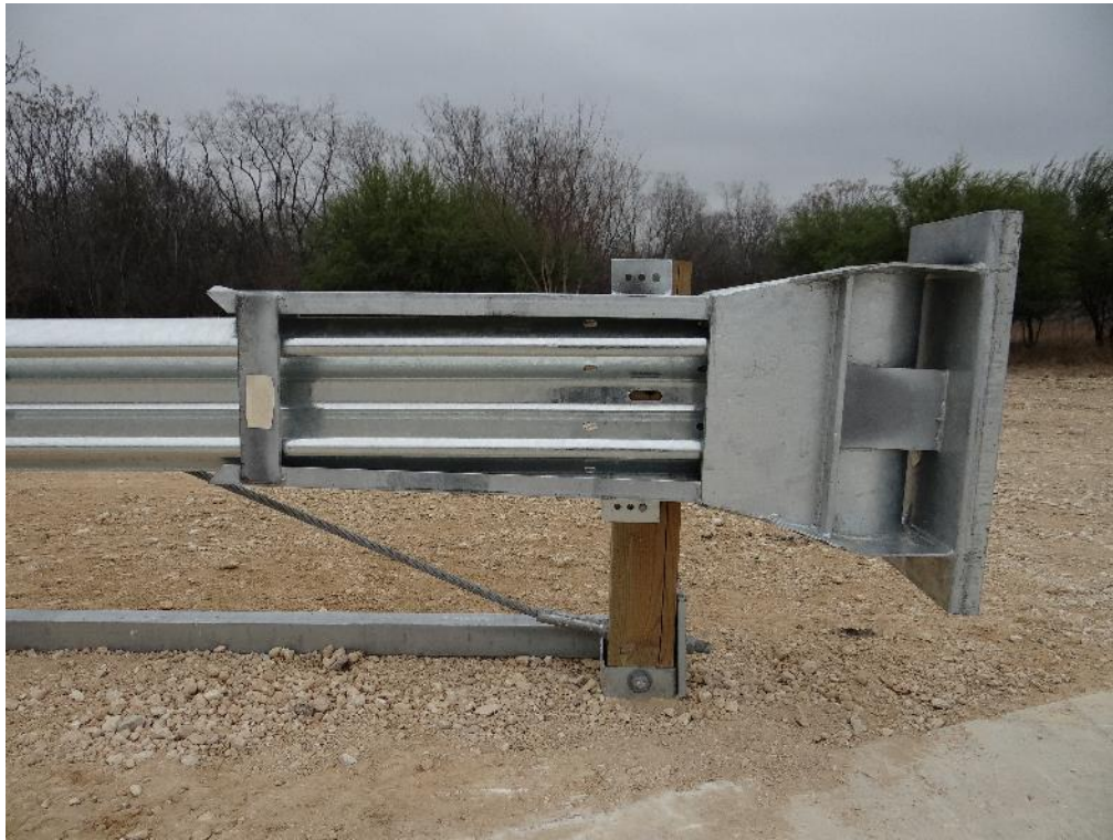
Figure 2.15: ET Plus Head and Post 1 – Traffic Side
