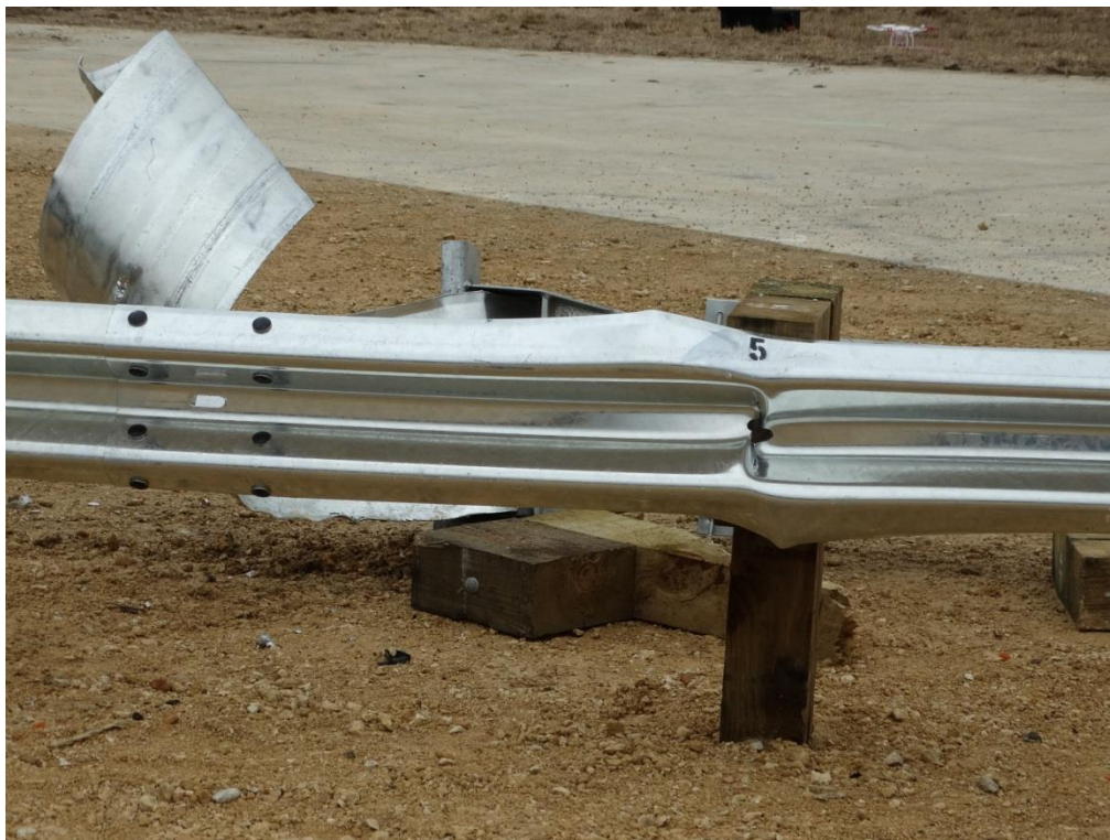
Figure 3.15: Post Test – Post 5, Traffic Side View
