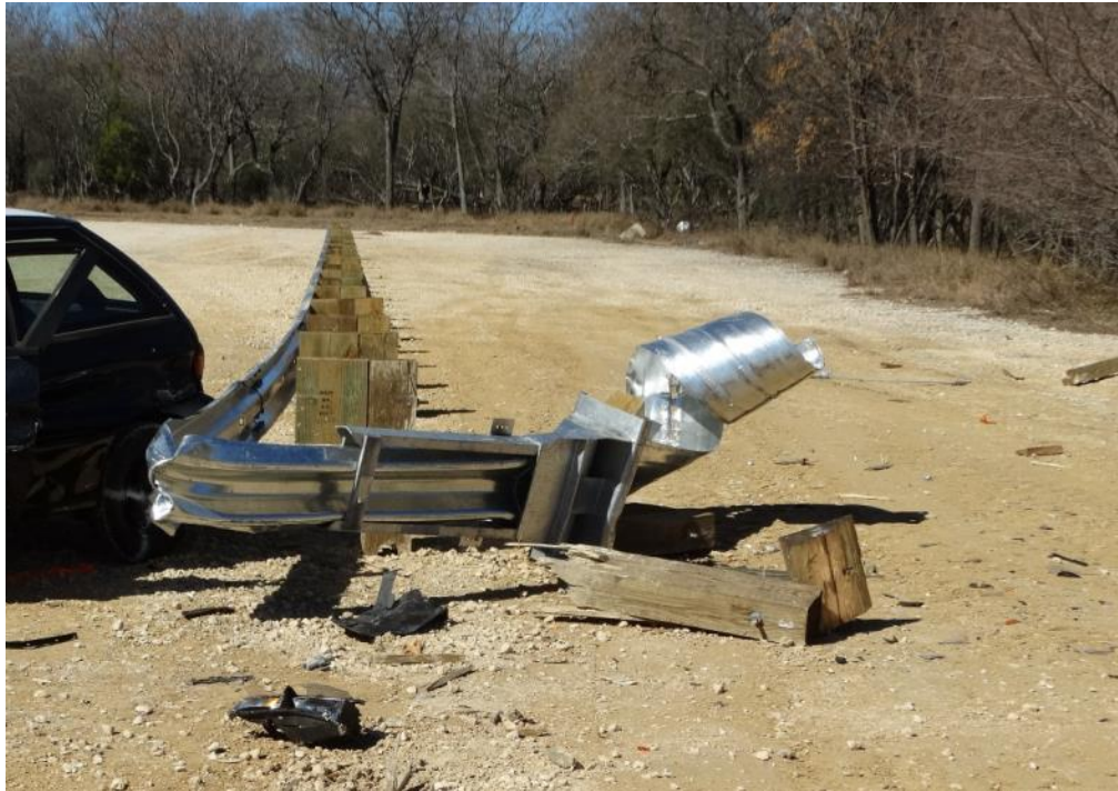
Figure 3.9: Post Test – Downstream Traffic Side View of Extruder Head
