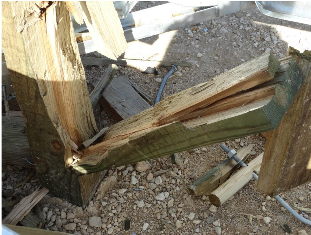
Figure 3.14: Post Test – Post 9 Damage
