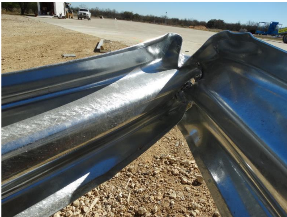
Figure 3.30: Post Test – Non-Traffic Side View of Folded W Beam at Post 4
