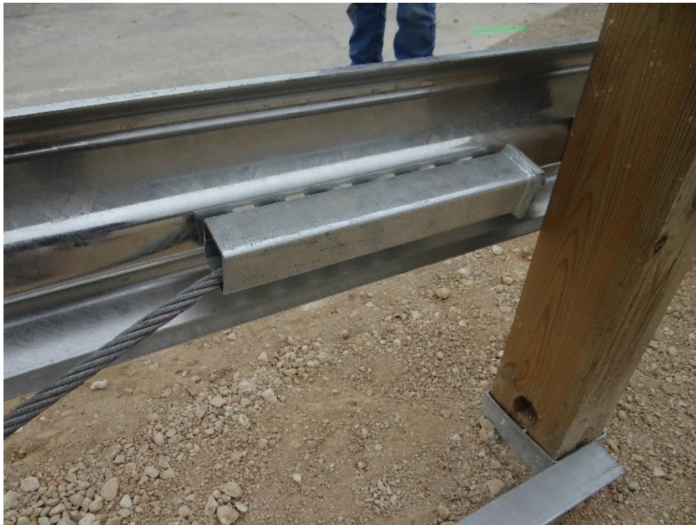
Figure 2.10: End Terminal Cable Anchor at Downstream End
