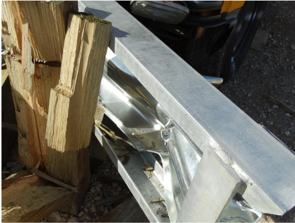
Figure 3.32: Post-Test – ET Plus Head, Non-Traffic Side, Close-up
