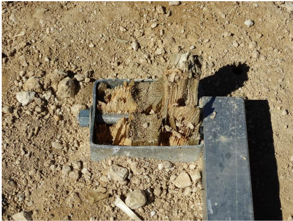
Figure 3.17: Post Test – Foundation Sleeve at Post 2
