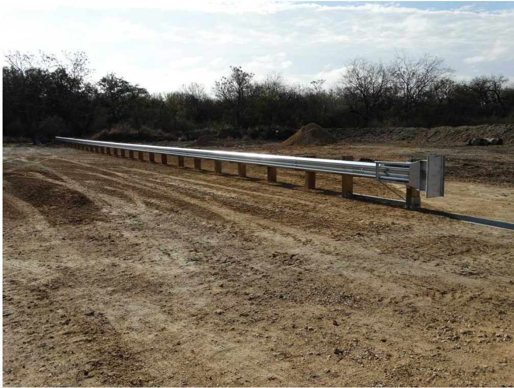
Figure 2.3: Test Installation for ET Plus Test ET31-31
