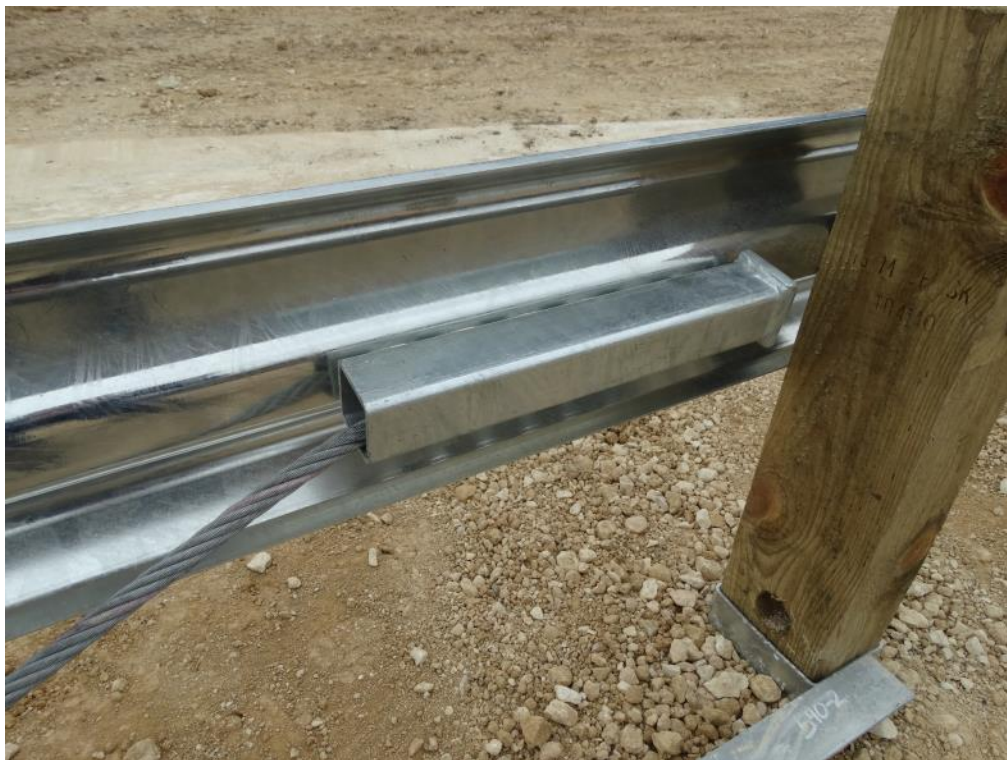
Figure 2.10: End Terminal Cable Anchor at Downstream End
