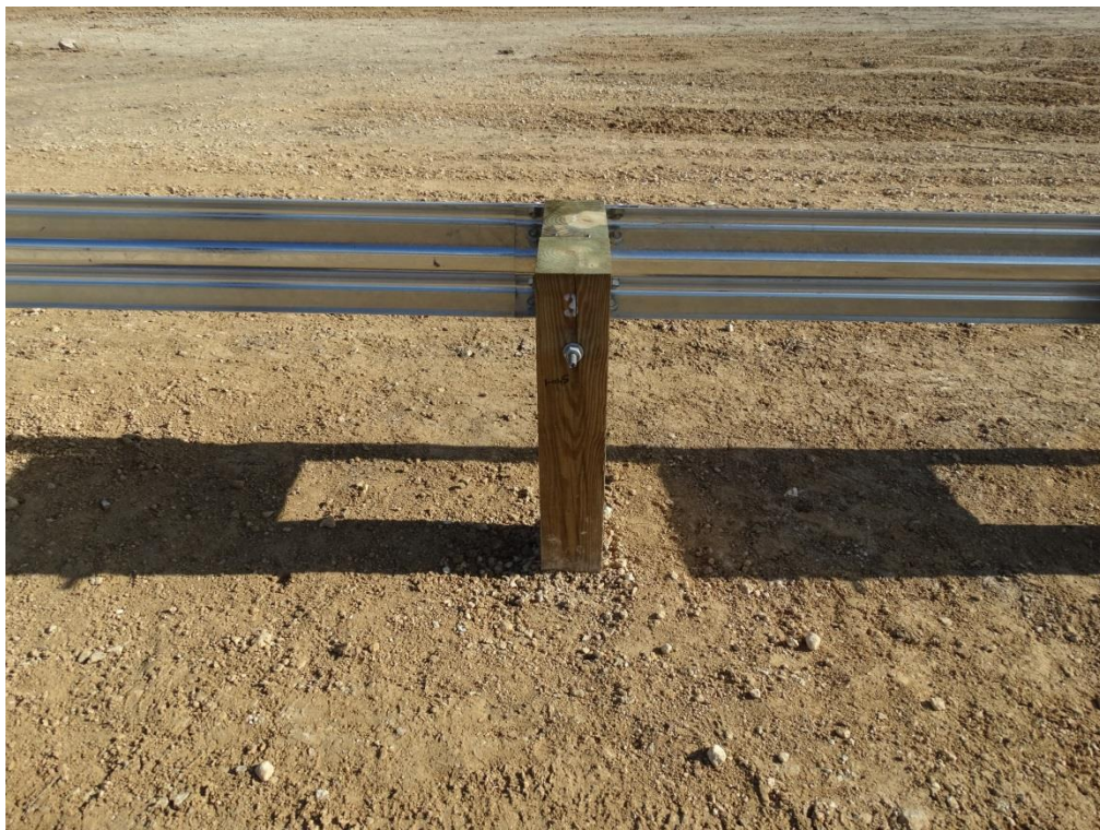
Figure 2.12: First Guardrail Panel Splice Joint – Non-Traffic Side
