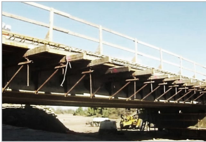
Gila River Slide-In Bridge
