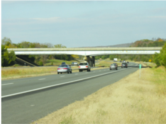
Side View of Rt. 15 over I-66 Bridge in Haymarket, Virginia
