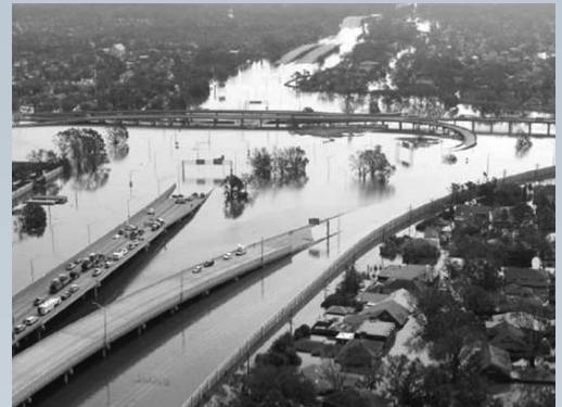
New Orleans, LA - East-bound I-10 near the I-90 interchange.
