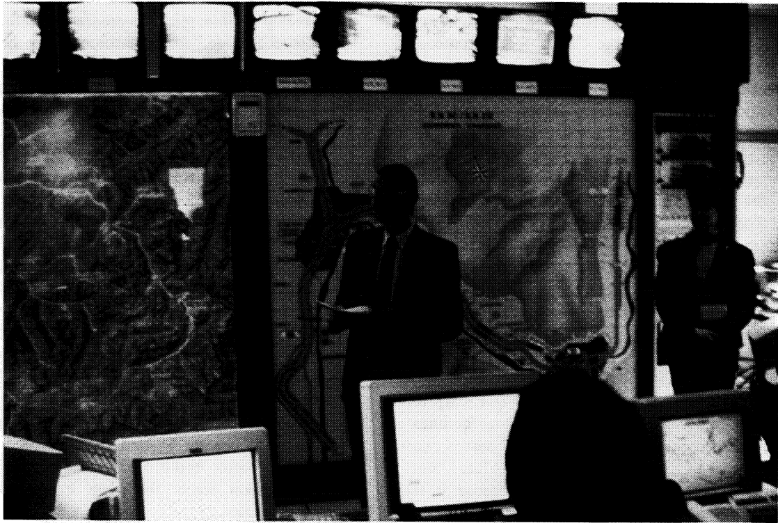
Figure 8. OSIRIS TMC Control Center.
