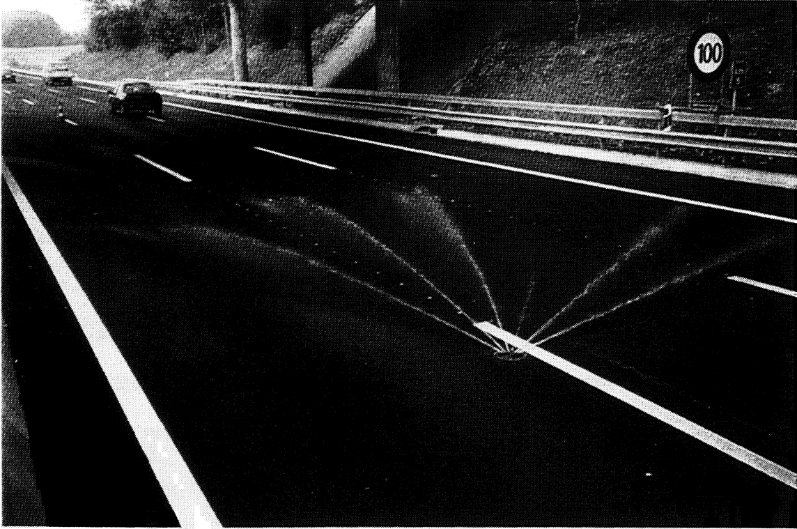
Figure 6. Spray head in action, automated salt spraying system, Lausanne, Switzerland.
