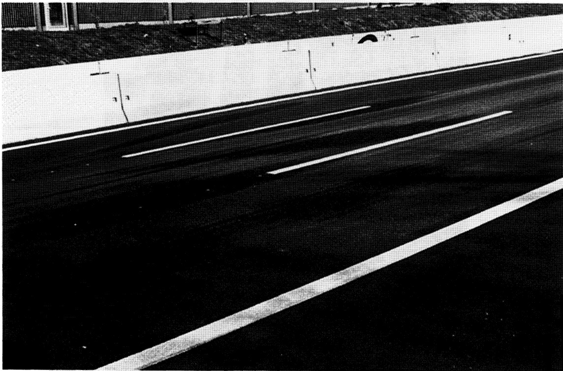
Figure 7. Salt residue on pavement after earlier activation of automated salt sprayers.
