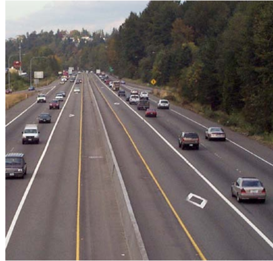
Pre-express toll lanes: SR 167 had two general purpose lanes and one HOV lane.
