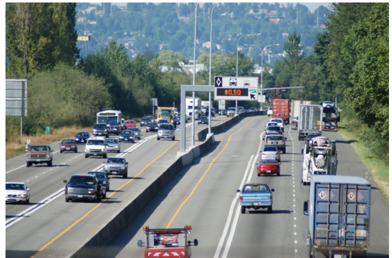
Post express toll lanes: HOV lanes were converted to a single express toll lane in each direction.
