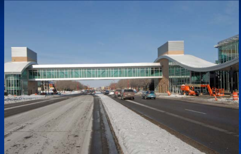
Apple Valley BRT Station
