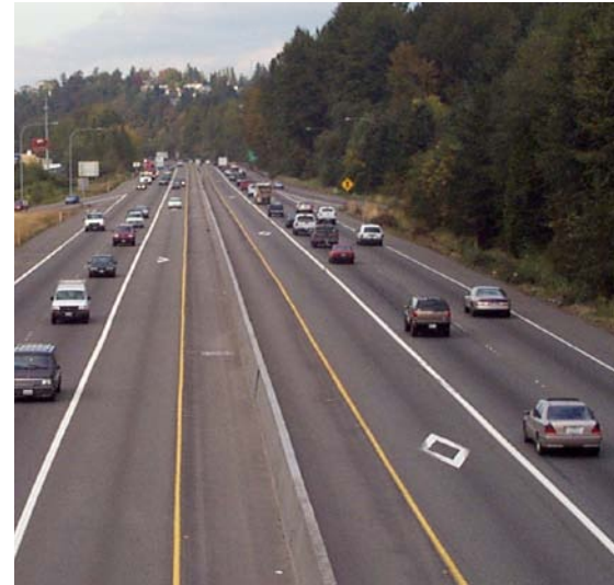
Pre-HOT lanes: SR 167 had two general purpose lanes and one HOV lane.
