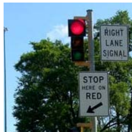
Figure 6-2: Ramp metering (Source: Wikimedia Commons/Patriarca12 2013)
