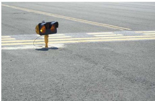
Figure 2. Example of Improved Airfield Lighting: Picture of an Elevated Runway Guard Light at Boston Logan
