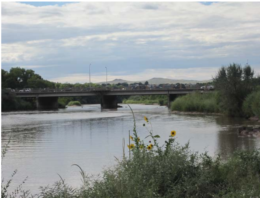
Figure 38: A Crossing of the Rio Grande River. Source: FHWA.
