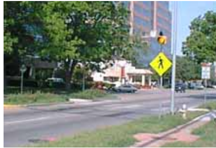
Figure 11-5. Photo. Fluorescent yellow-green sign treatment in Austin, TX.
