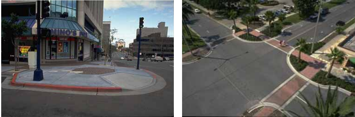
Figure 11-10. Photos. Curb extensions reduce crossing distances for pedestrians and provide additional corner storage space.
