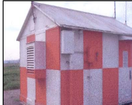
Figure 9. Power Shed at Long Beach Airport
