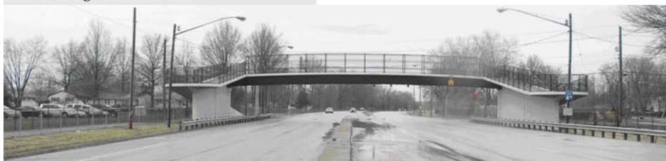
RSA finding: Hidden Traffic Signal
