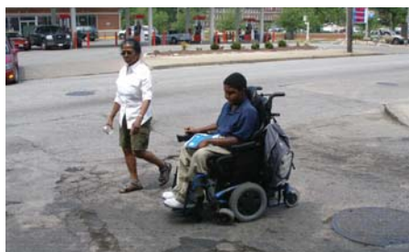
RSA finding: Lack of Pedestrian Facilities
