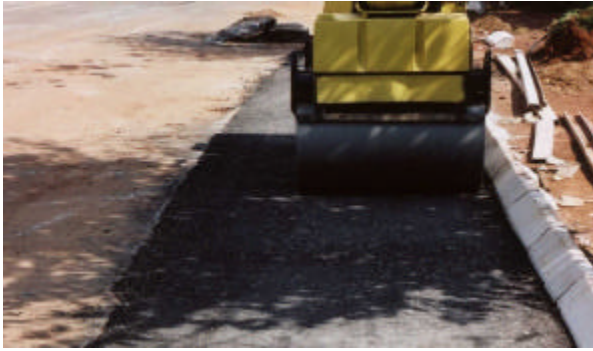
Figure 9. Vibratory compaction of FTBC
