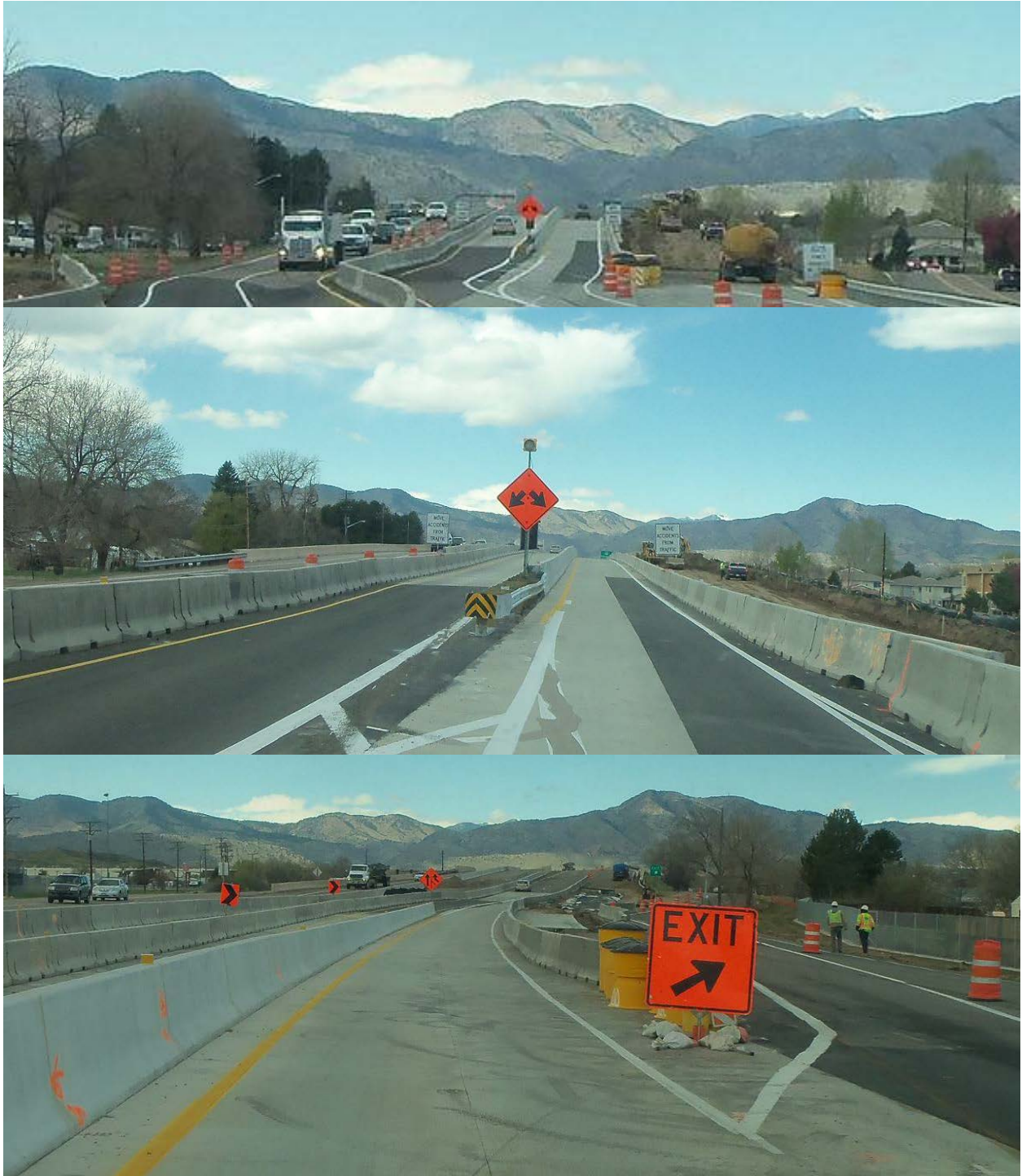
Figure 4-6. Barrier Separated Through Lanes on Westbound US 285 (Top: in advance of lane separation; Middle: at separation; Bottom: at Kipling off-ramp)
