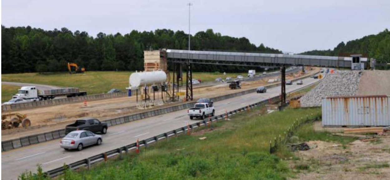
Figure 6-2. I-40 Widening Project Material Conveyor
