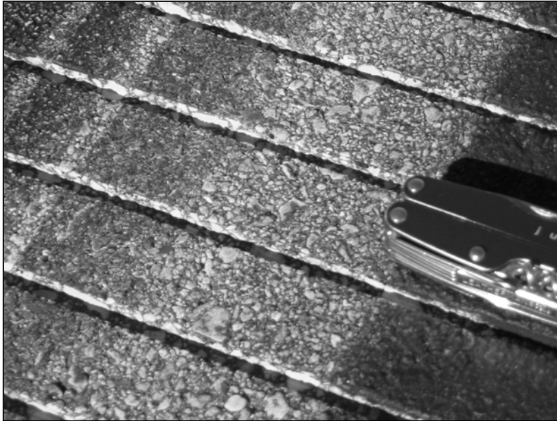
Figure 6—Grooving on Superpave Runway at Volk Field after 4 Years (Courtesy Erv Dukatz)
