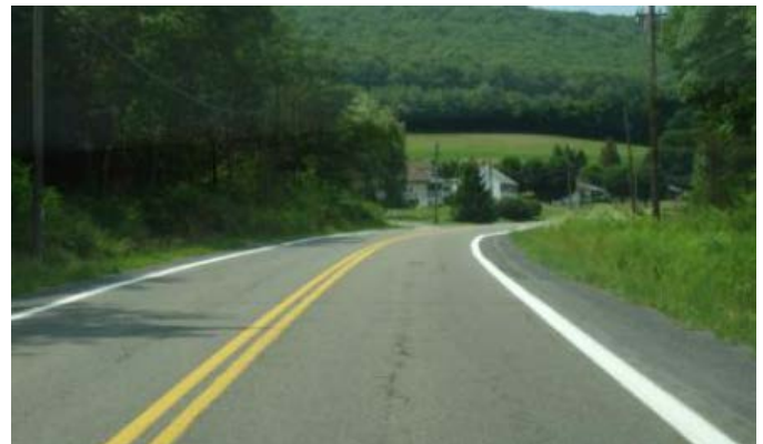
Rural Roadway Featuring 8-inch Edge Line (Photo courtesy of FHWA)
