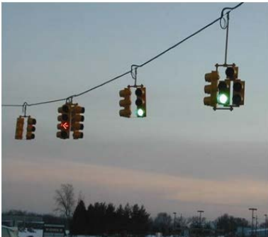
Photo courtesy of FHWA
