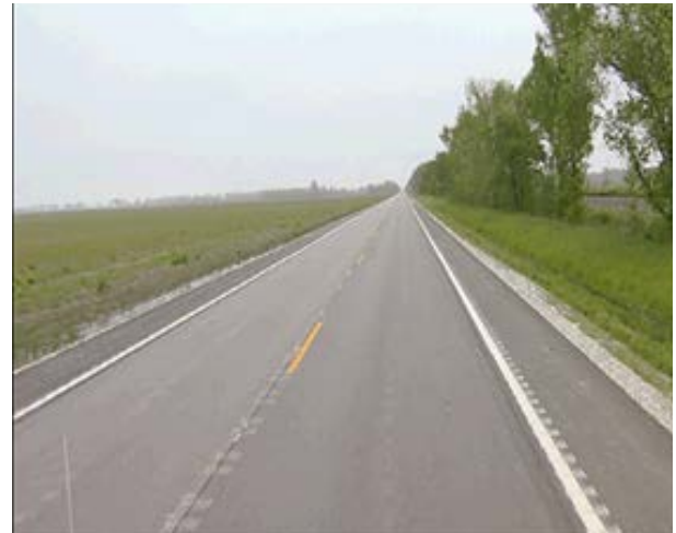
Edgeline and centerline striping are combined with wide shoulders to combat lane departure crashes in Missouri. (Photo courtesy of Missouri DOT.)
