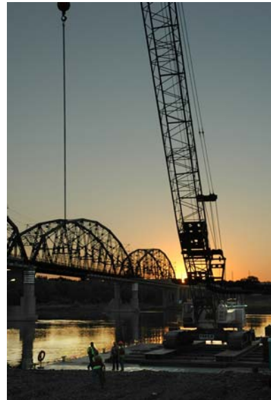
Liberty Memorial Bridge, Bismarck
