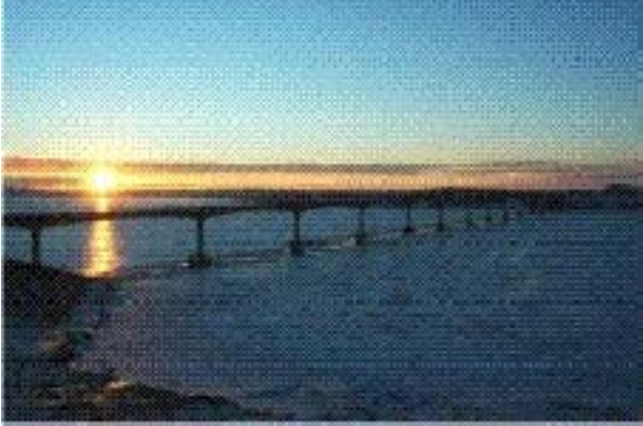
Four Bears Bridge, New Town
