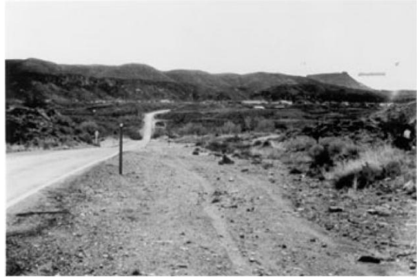
Typical Roadway with Roadside Hazard Rating Equal to 2.
