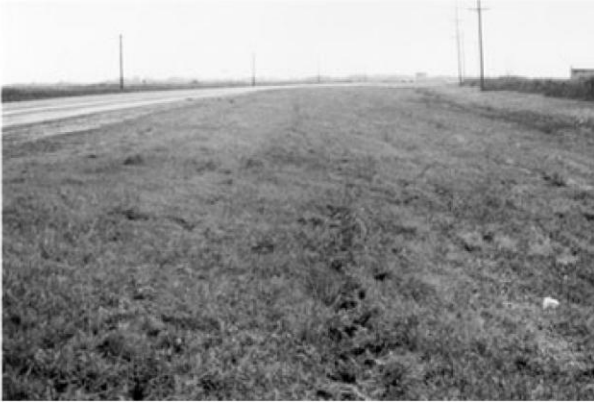
Typical Roadway with Roadside Hazard Rating Equal to 1.
