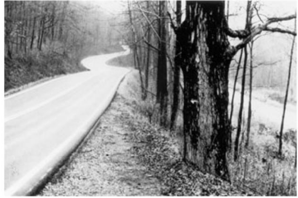
Typical Roadway with Roadside Hazard Rating Equal to 6.
