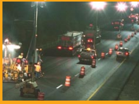
Improving Traffic Control for Night Work Zones
