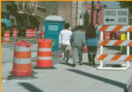
Accommodating Pedestrians in Work Zones
