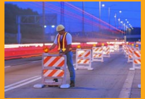
Worker Safety and Visibility
