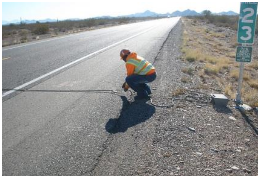
Continuous Count Station (source: AZ DOT )
