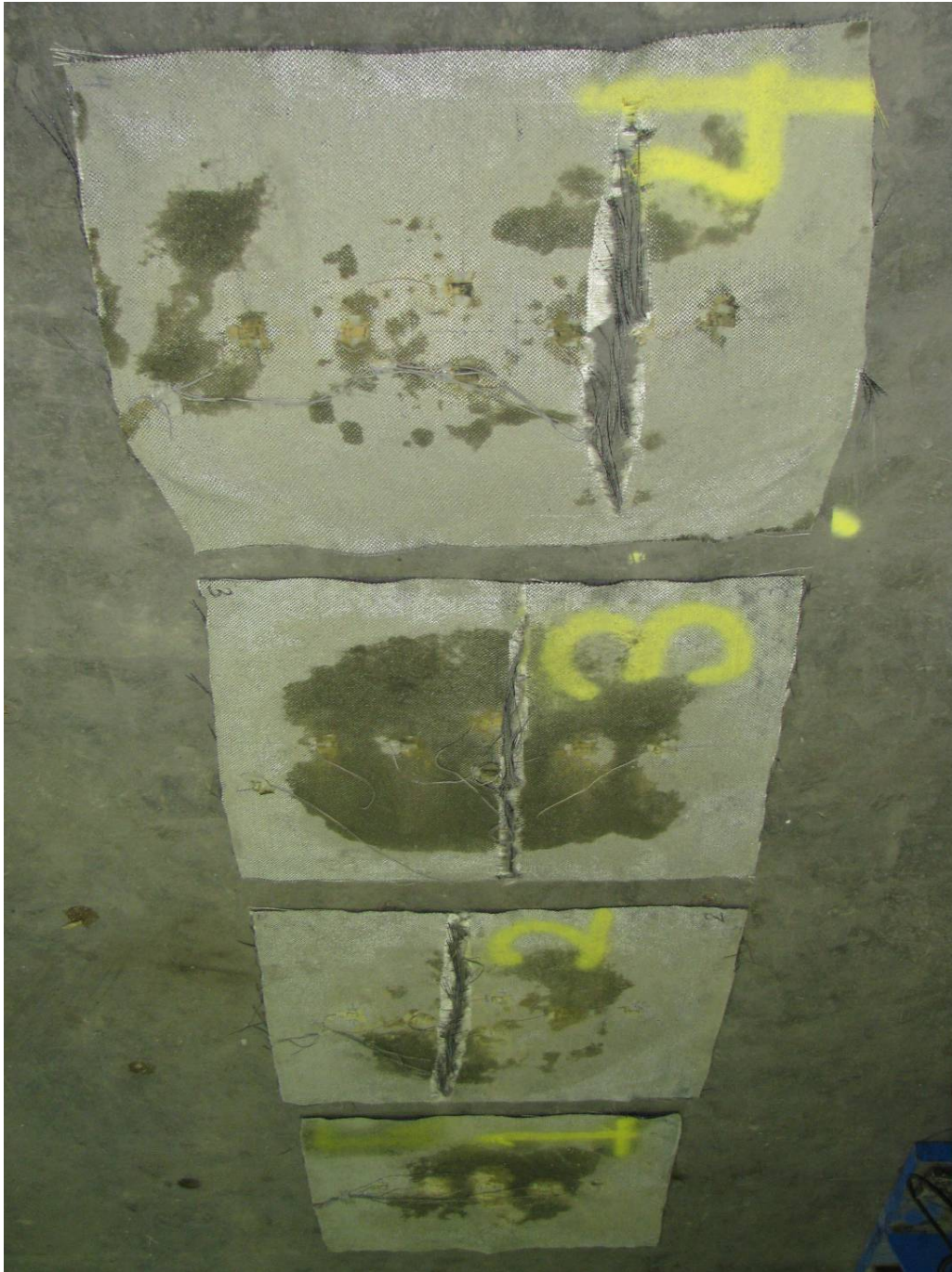
Figure 175. Photo. Aerial view of the reinforcement sheets exhumed from the composite mass after test 3 (numbers indicate sheet number).
