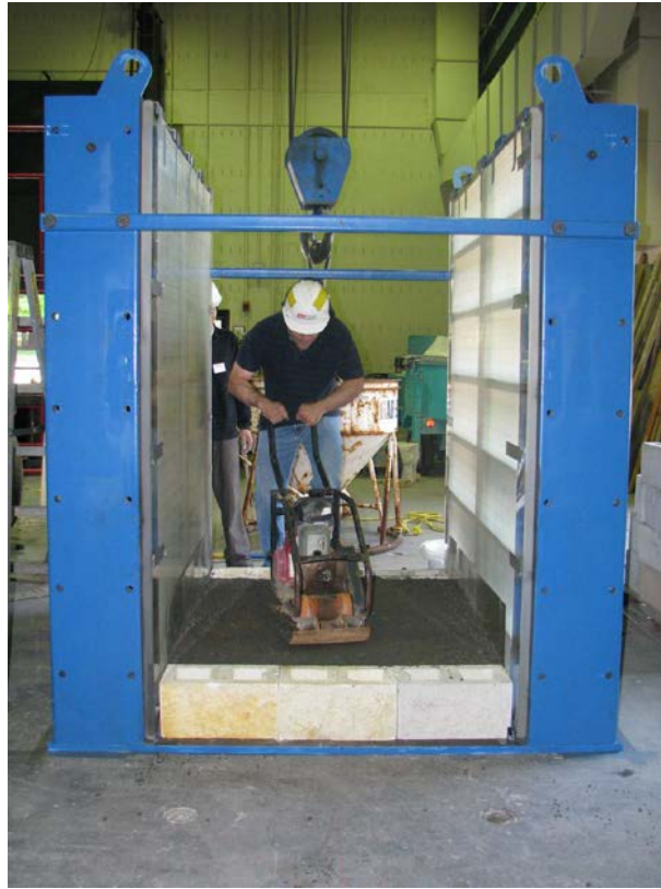
Figure 128. Photo. Compacting the first lift of backfill.
