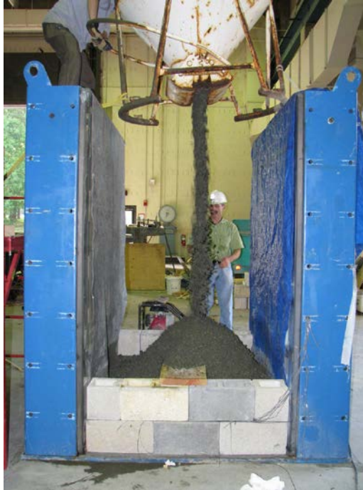
Figure 129. Photo. Placing backfill for the second lift.
