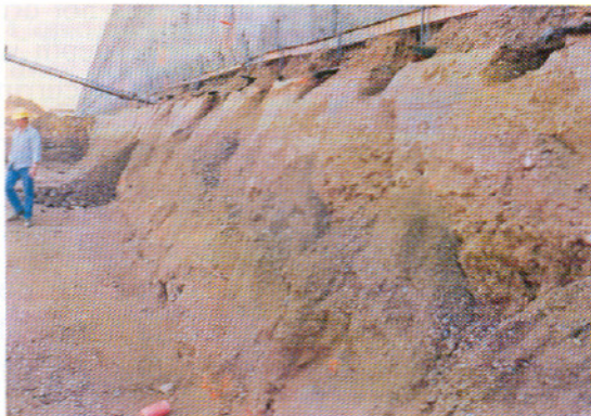
P47. Drilling through stabilizing berm.
