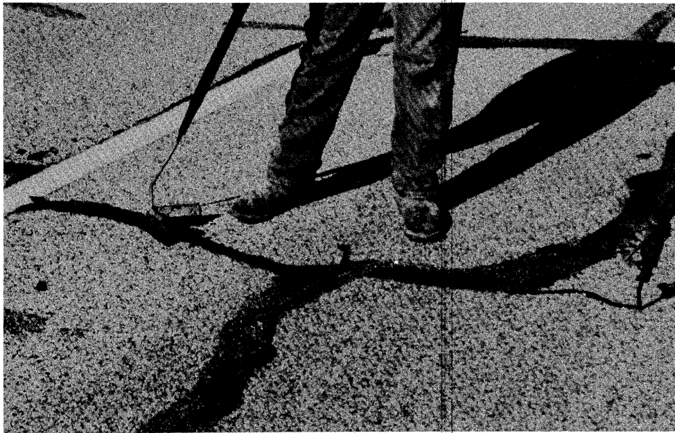
Figure 44. Finishing and shaping the sealant using hand squeegee.
