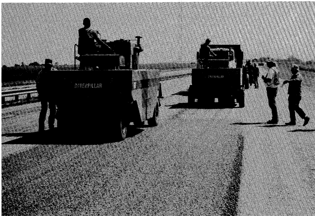
Figure 20. Compacting chip seals using rubber wheel rollers.
