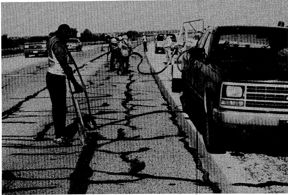
Figure 43. An asphalt kettle with pressure applicator.
