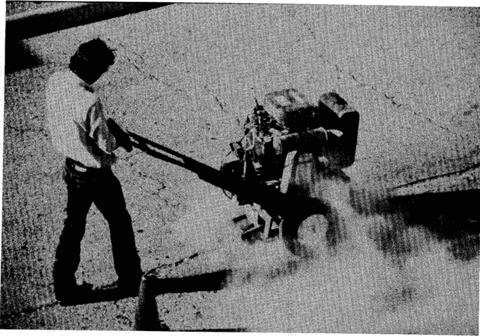
Figure 41. Router for shaping cracks.
