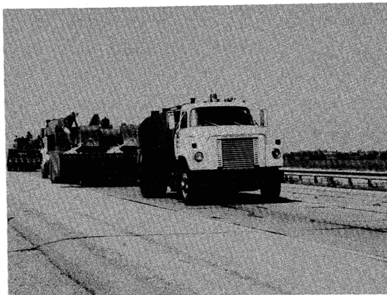
Figure 18. Asphalt distributor, chip spreader and rollers.
