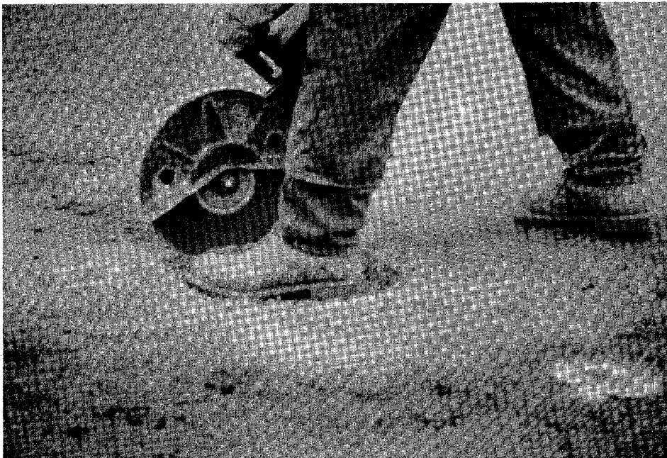
Figure 6-2. Pavement saw cutting semi-permanent repair boundaries.
