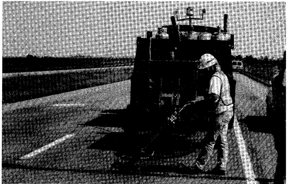
Figure 5-7. Hot airblasting using HCA (heat) lance.
