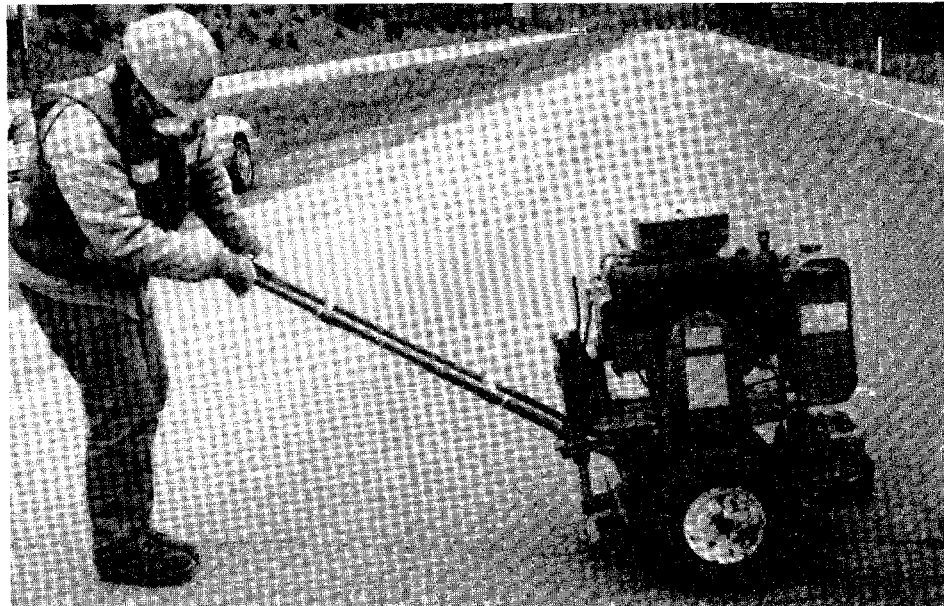
Figure 5-5. Routing with a rotary-impact router.
