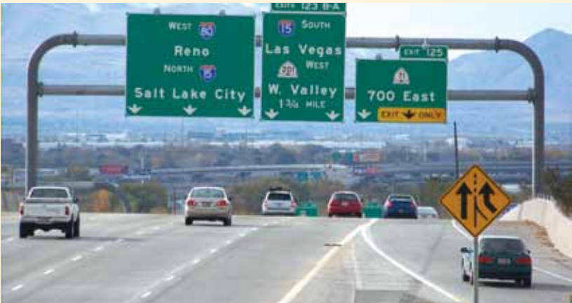
Well maintained overhead signs on a protected concrete structure at the junction of I-15 and I-80 in Salt Lake City and a merge sign with slip base that makes replacement easier and safer for the maintenance crew.
