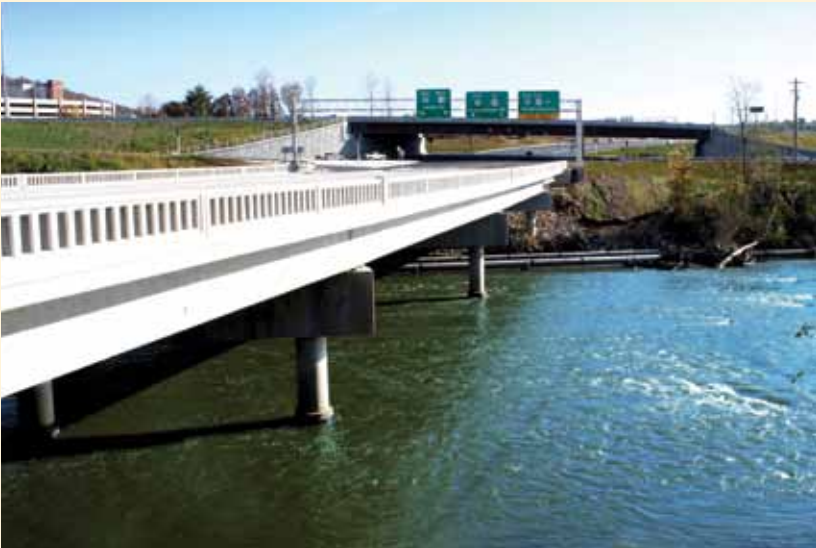
New bridge at I-26 Interchange with NC 146 in Asheville
