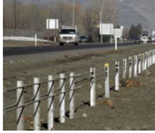
Figure 32. Photo. Barrier type 7—high-tension cable guardrail system. (15)
