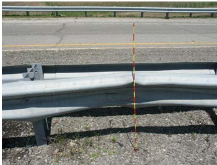
Figure 23. Photo. Photograph from Case No. 2005073438121 in which measurements were obtained using rods.
