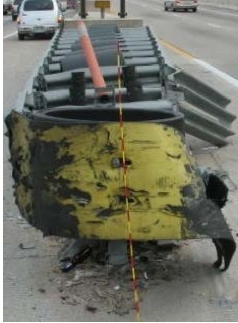
Figure 45. Photo. Barrier type 19—impact attenuator. (4)
