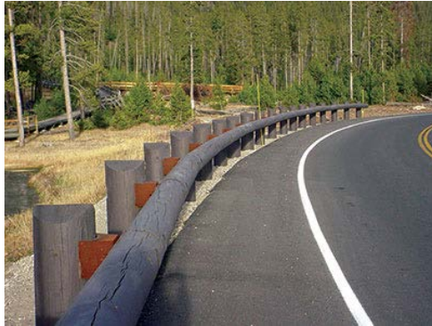
Figure 24. Photo. Barrier type 1—esthetic timber barrier/wood guardrail. (17)
