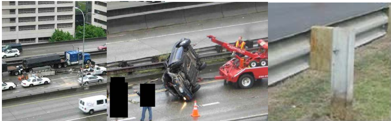
Figure 16. Photo. Case No. 2005082626081 post-crash impact attenuator (left) in advance of W-beam strong post (center) contrasted with comparative catalog image (right). (4,14)
