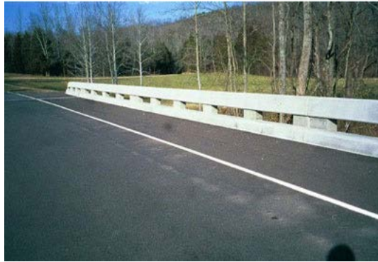
Figure 27. Photo. Barrier type 3—bridge rail. (20)
