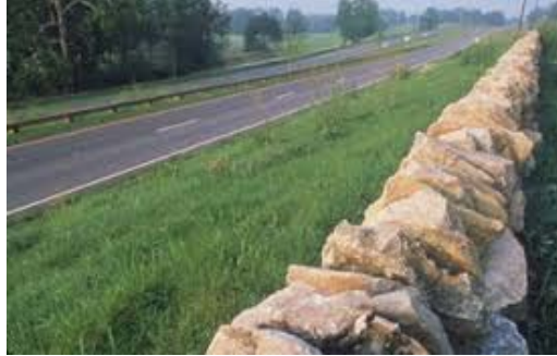
Figure 51. Photo. Barrier end treatment type 3—rock fence. (26)
