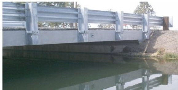
Figure 39. Photo. Barrier type 13—Thrie beam. (20)
