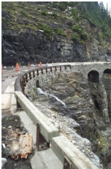
Figure 25. Photo. Second image of barrier type 1—esthetic timber barrier/wood guardrail. (18)
