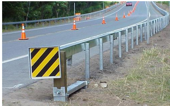
Figure 43. Photo. Barrier type 17—weak post box beam. (23)
