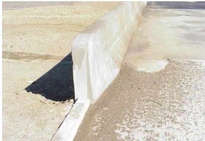
Figure 34. Photo. Second image of barrier type 8—Jersey barrier. (20)
