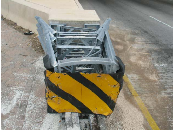
Figure 58. Photo. Barrier end treatment type 12—temporary impact attenuators. (4)
