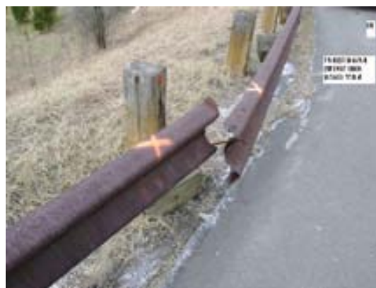
Figure 44. Photo. Barrier type 18—weathering steel (Corten®) guardrail. (14)
