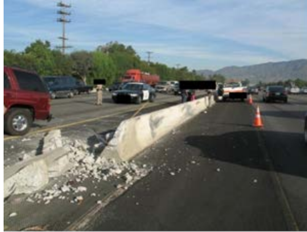
Figure 8. Photo. First view of Case No. 2005079486822 showing the point of impact.
