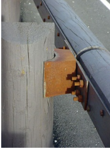
Figure 38. Photo. Barrier type 12—steel-backed timber guardrail. (17)
