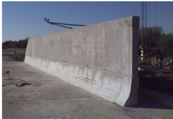
Figure 31. Photo. Barrier type 5—F-shaped barrier. (20)
