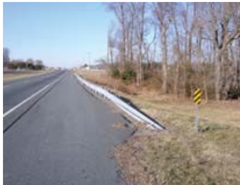
Figure 53. Photo. Barrier end treatment type 6—“turndown” roll-over end section. (14)
