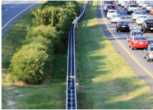
Figure 36. Photo. Barrier type 10—median barrier steel guardrail. (15)
