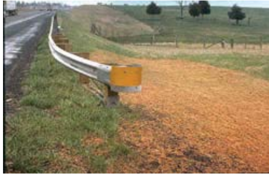
Figure 42. Photo. Barrier type 16—W-beam weak post. (14)
