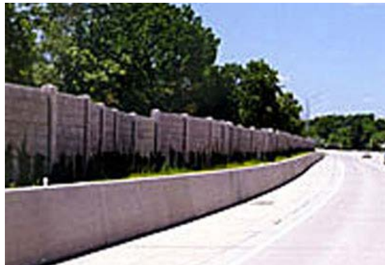
Figure 30. Illustration. Barrier type 4—constant slope barrier. (20)
