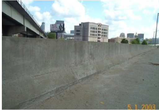
Figure 33. Photo. Barrier type 8—Jersey barrier. (20)
