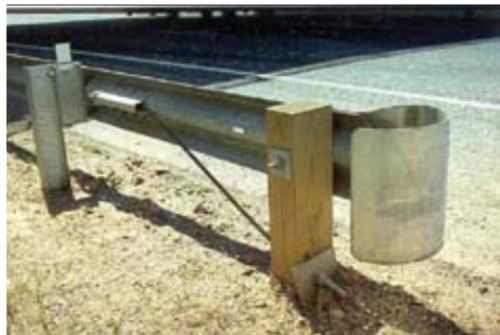
Figure 52. Photo. Barrier end treatment type 4—rounded terminal buffer (“question mark”). (14)
