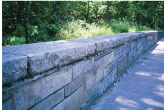
Figure 28. Photo. Second image of barrier type 3—bridge rail. (20)
