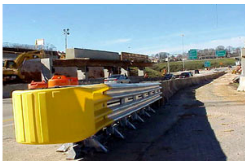
Figure 57. Photo. Barrier end treatment type 12—impact attenuators. (27)
