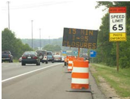
Figure 47. Photo. Third image of barrier type 19—impact attenuator. (24)
