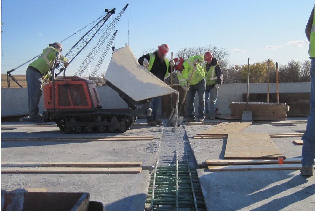
Figure 1. Photo. Casting of a grout-type material in the connections between PBEs.
