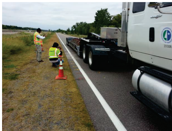
Figure 35. Photo. Verifying the embedded sensor alignment.
