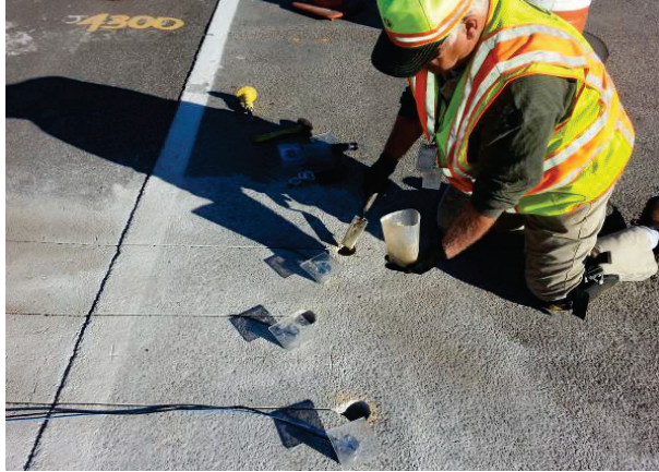
Figure 28. Photo. Partial grouting of the sensors.
