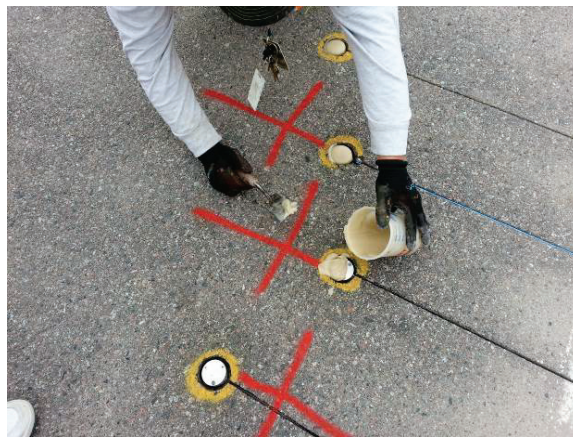
Figure 34. Photo. Final grouting of sensors.
