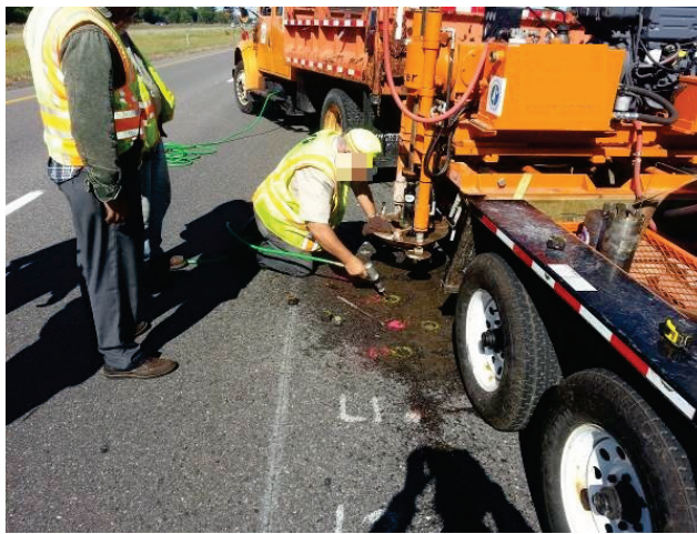
Figure 26. Photo. Smoothing of holes for sensor installation.
