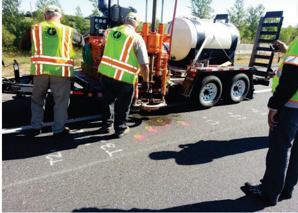
Figure 25. Photo. Pavement coring for sensor installation.
