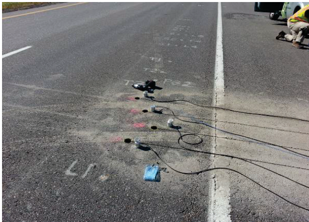
Figure 27. Photo. Grooving of pavement for sensor installation.
