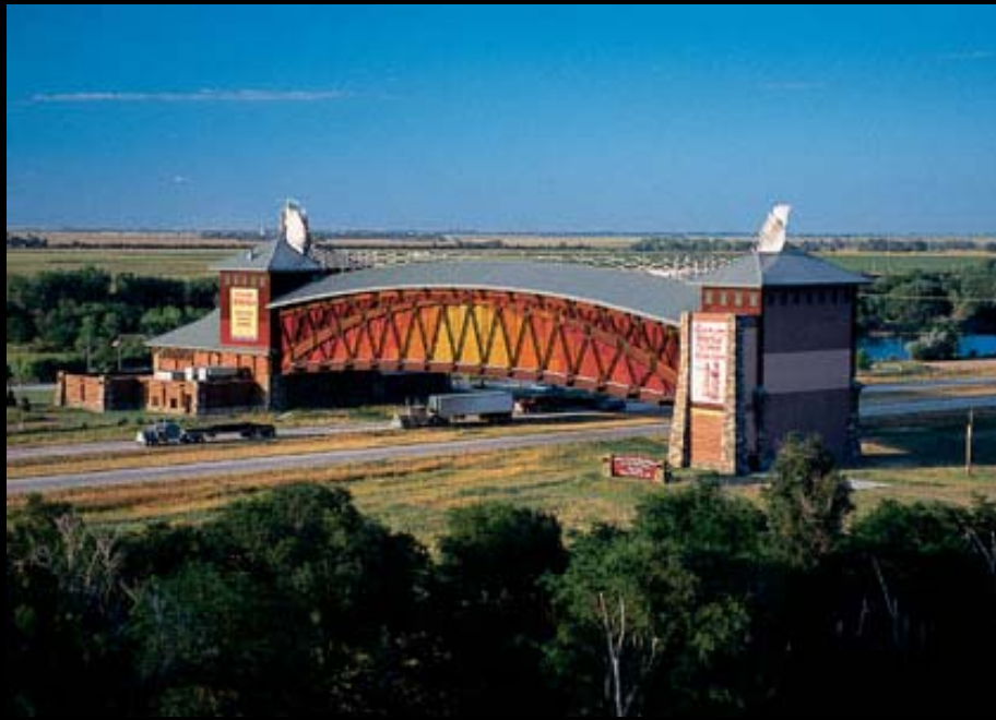
Towering over Interstate 80, the Great Platte River Archway Monument near Kearney delivers a one-of-a-kind interactive experience. TITLE: Arch BY: J. Nabb
