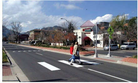
A center island raised median.
