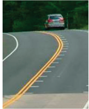
Optical speed bars on a rural roadway placed in advance of a horizontal curve.
