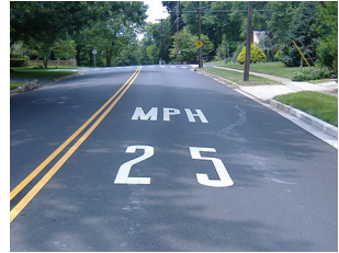
Special pavement marking to encourage speed reduction for impending curve.
