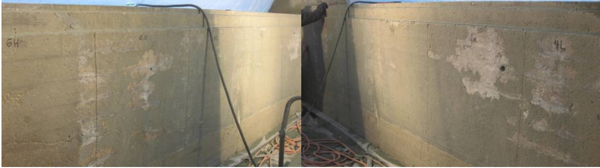
Figure 4.32: The bridge sections before anode removal by: (left) #6 nozzle; (right) #4 nozzle.
