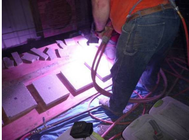
Figure 4.12: Arc-spraying the PCC samples.
