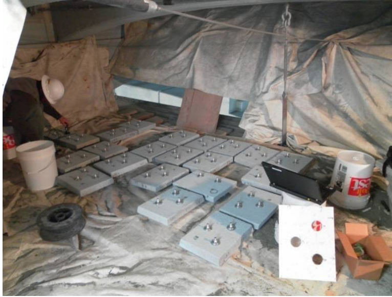
Figure 4.30: PCC and mortar samples being bond tested.
