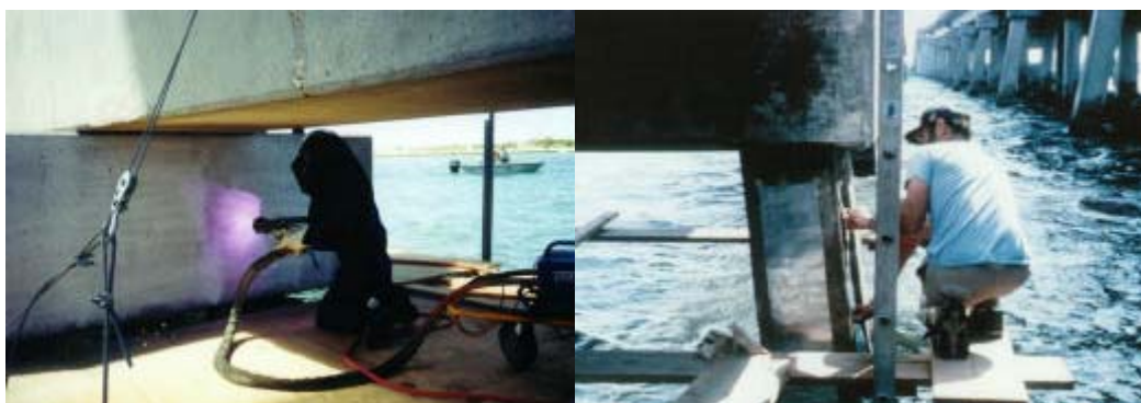
Figure 2.2: Arc spray application of galvanic Al-Zn-In to a bridge pier in Texas (left); and application of zinc/hydrogel anode to a bridge pier in Florida (right) (Daily 1999).
