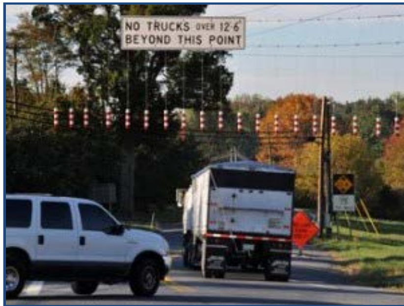
Figure 49. Photo. Truck Over-Height Warning System. (8)
