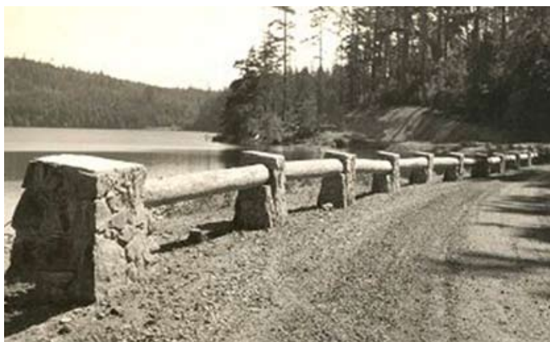
Constructed by Civilian Conservation Corps (CCC) workers during the Great Depression, the original log rail barriers in Deception Pass State Park are of historic significance due to their age, quality of workmanship, and context sensitive design.
