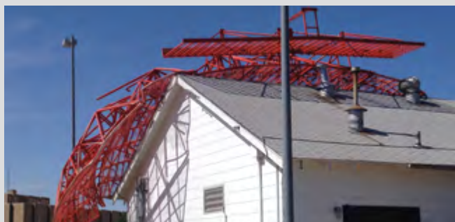
293 mph winds toppled a long-range radar antenna onto a building at the MMAC. Photo: FAA.
