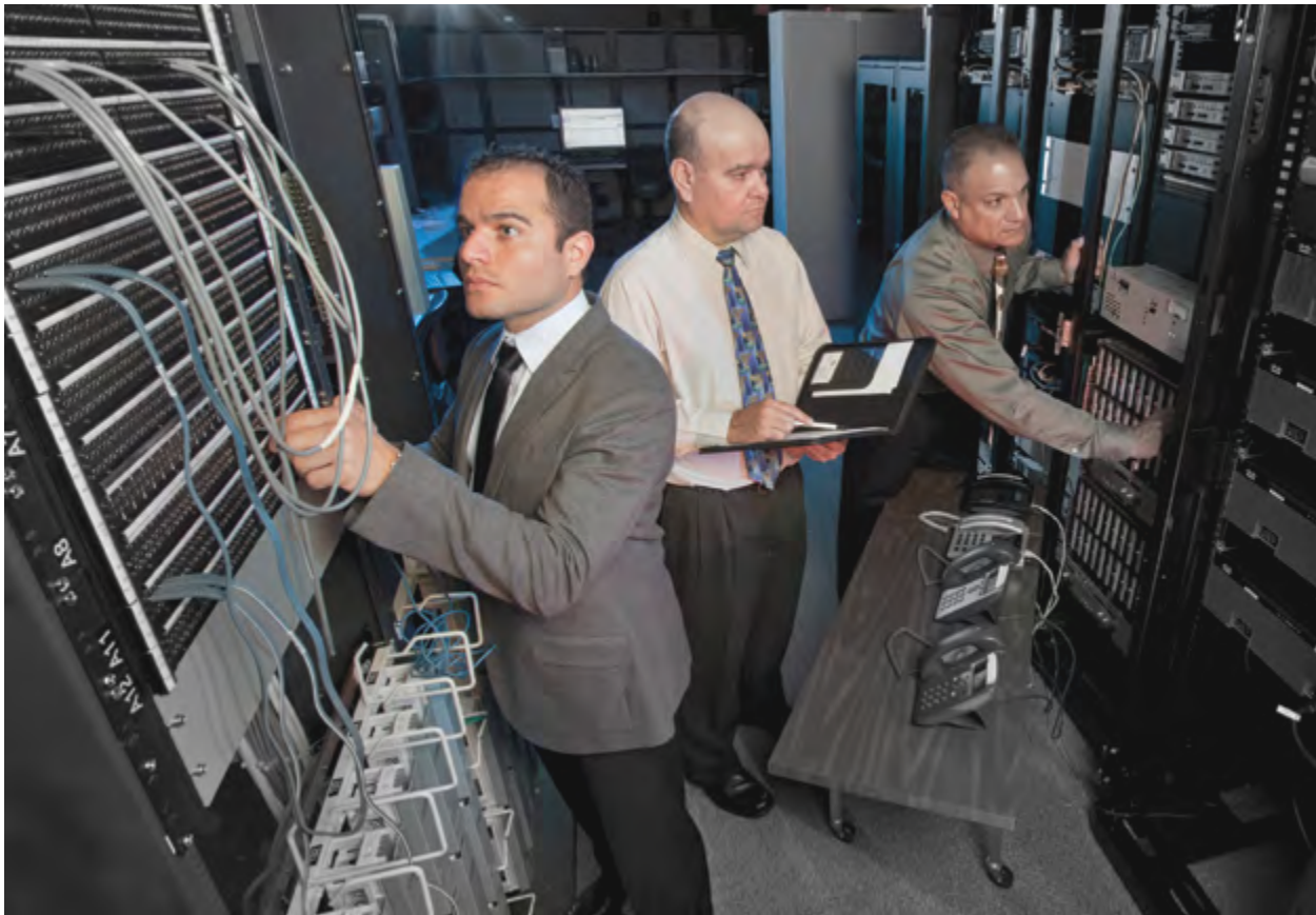
FAA personnel validating equipment installation prior to operational testing. Photo: FAA.
