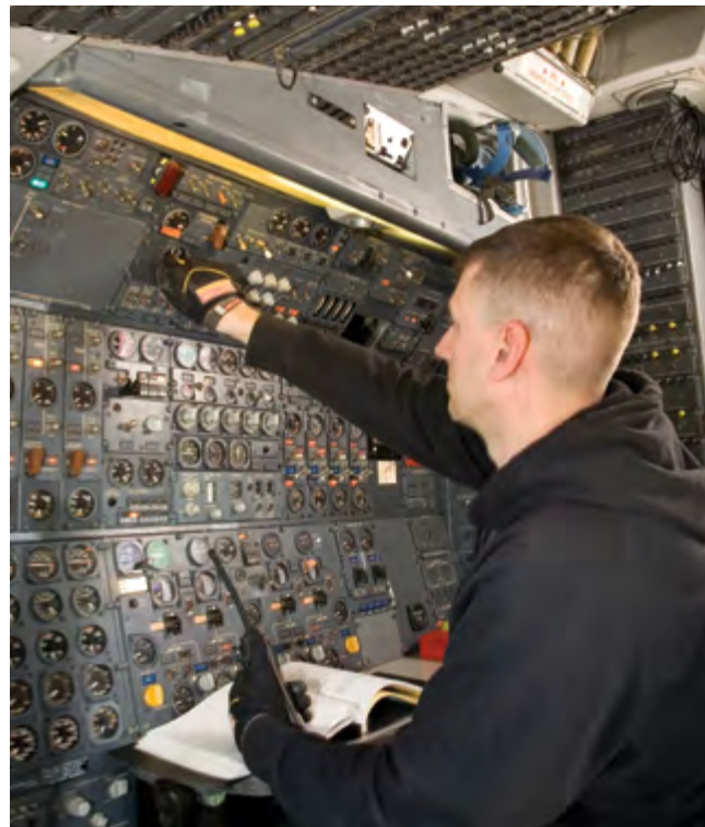
Cargo compartment smoke-detection testing. Photo: FAA.
