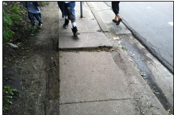
Figure 9: Heaved sidewalk
