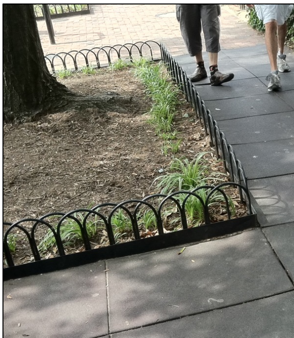
Figure 37: Modular plastic pavers near a tree.
