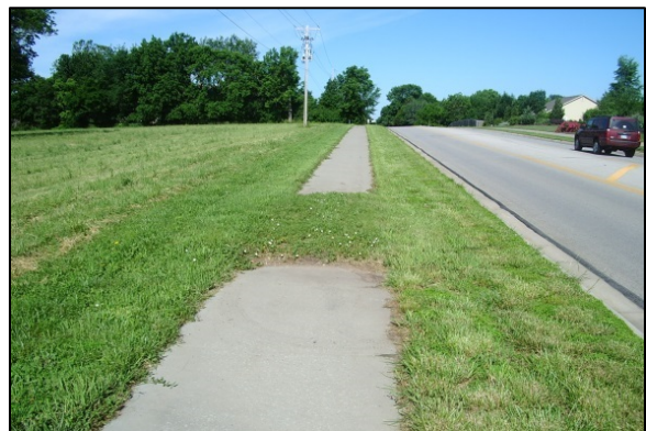
Figure 16: Soil accumulation across a sidewalk has allowed for thick vegetation overgrowth which limits the use of the sidewalk by people with some disabilities.
