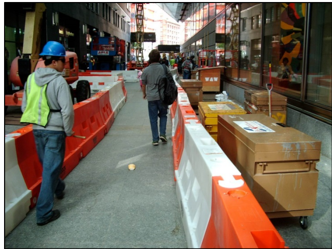
Figure 19: An accessible detour
