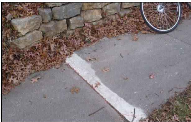
Figure 25: A raised sidewalk block has been ground down to provide a smoother transition.
