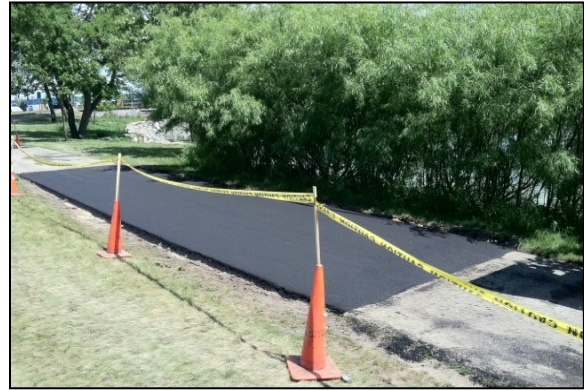
Figure 3: Asphalt is commonly used for shared use paths, but is less commonly used for sidewalks in the United States. Above is a section of shared use path after a repair in Madison, Wisconsin.
