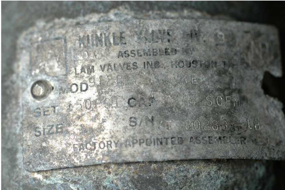
Figure 13: Shows PRD identified as 08H127-1
